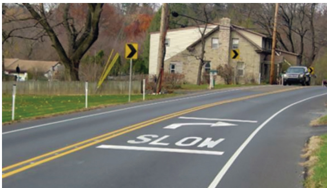
Figure 2. Delineation examples: pavement marking, chevron signs, and roadside delineation.
