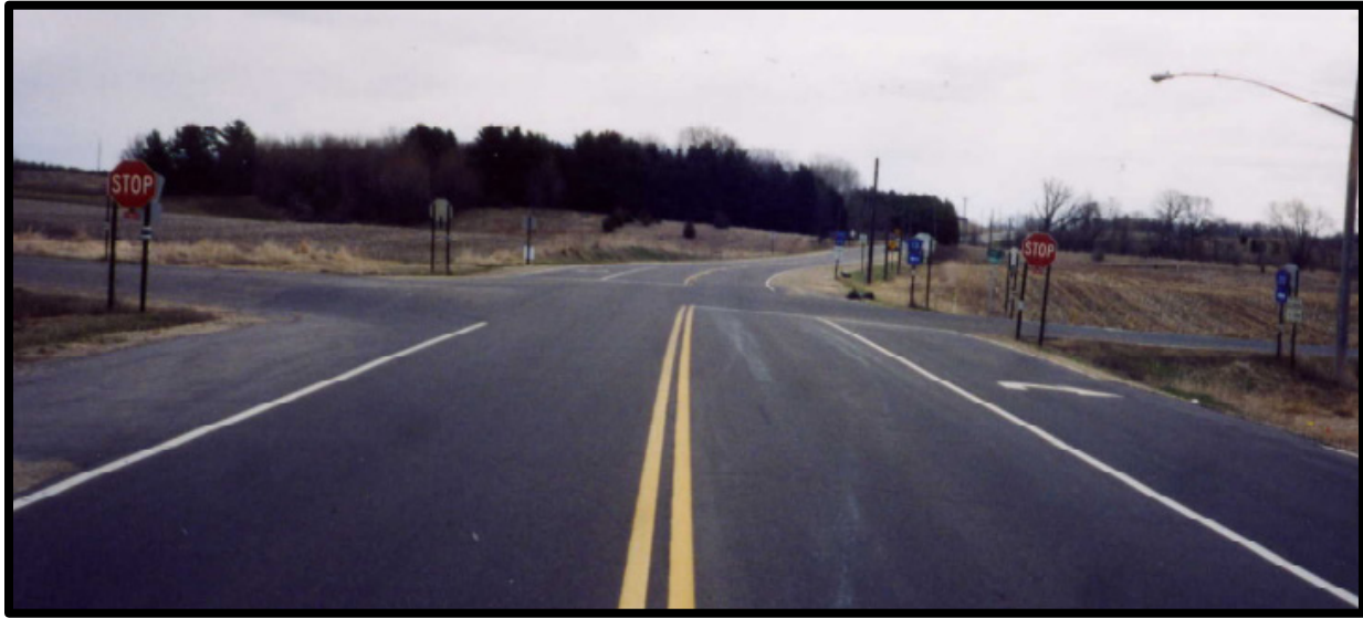
Figure 2 Intersection of County State Aid Highways 20 and 13 N in Washington County had no reported nighttime crashes during a three-year period following the installation of roadway lighting.
