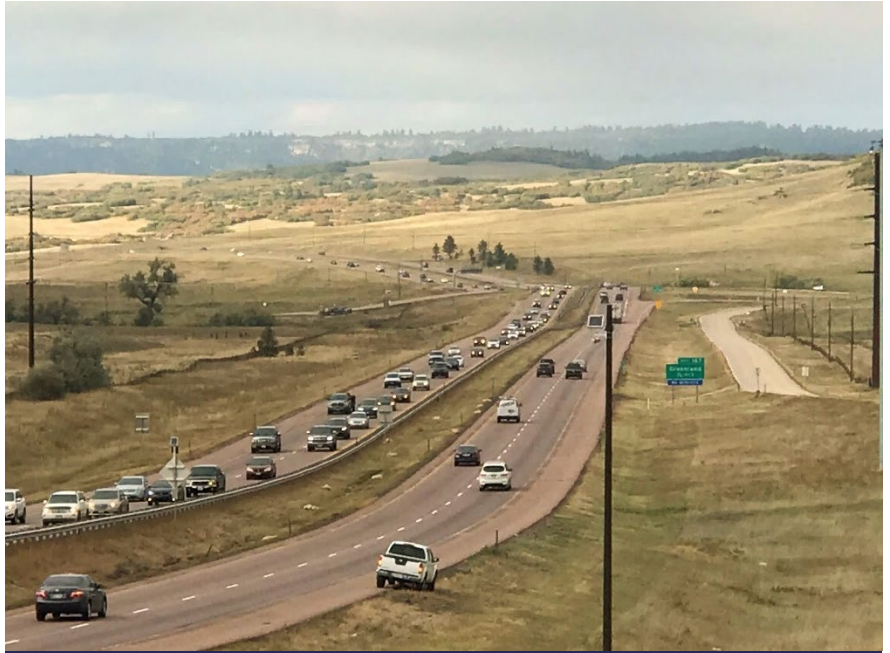
Figure 7. Photograph. Example of split grade and narrow shoulders in the Gap (2006-2016). Source: Attardo, 2020.
