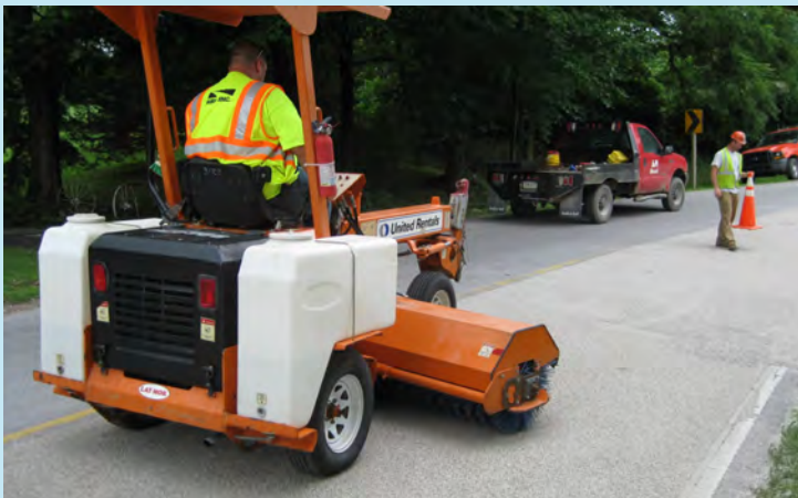
Figure 19. Photograph. Example of aggregate removal using a power broom.
