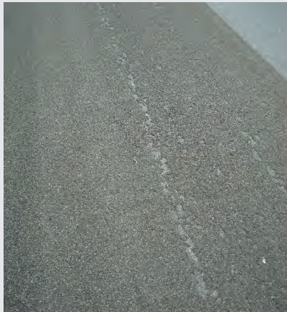
Figure 23. Photograph. Example of discoloration indicating uncured resin binder.
