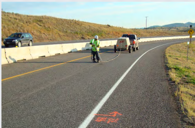
Figure 3. Photograph. Example of compressed air wash surface preparation.
