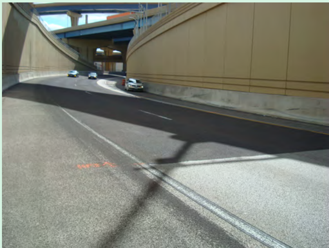
Figure 25. Photograph. Example of aggregate shedding and accumulation along lane edge and on paved shoulder.
