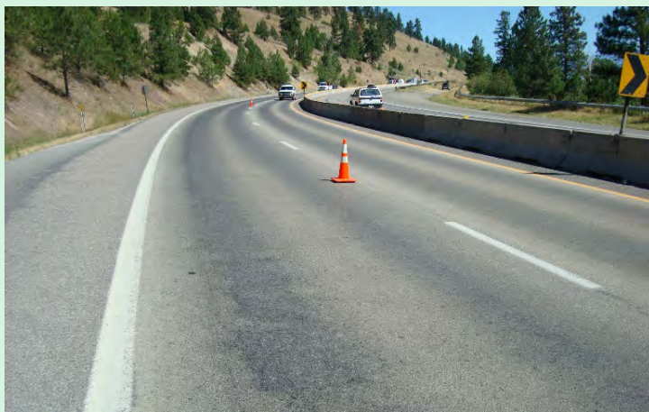
Figure 29. Photograph. Example of HFST worn off in the wheelpaths.
