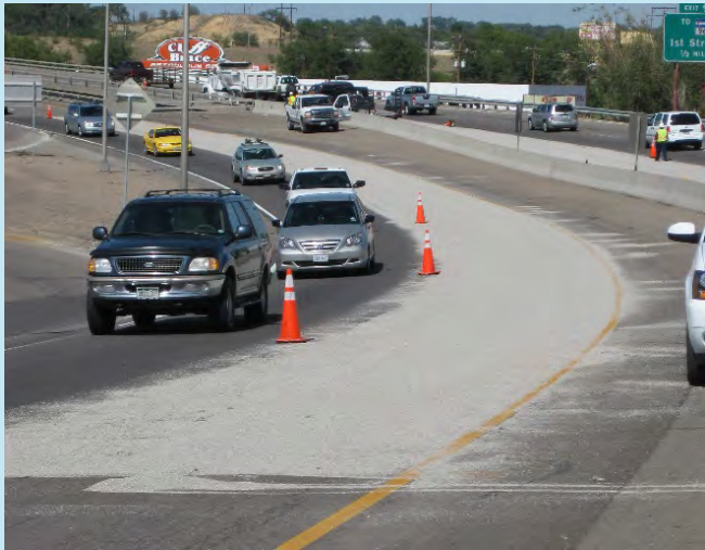
Figure 21. Photograph. Example of exposure of underlying pavement after sweeping.
