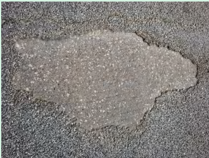
Figure 26. Photograph. Example of delamination of HFST from underlying pavement surface.
