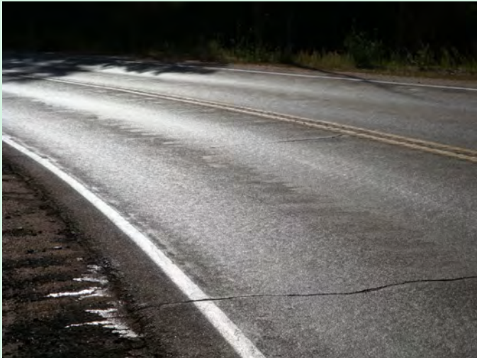
Figure 27. Photograph. Example of polished HFST surface in wheelpaths.
