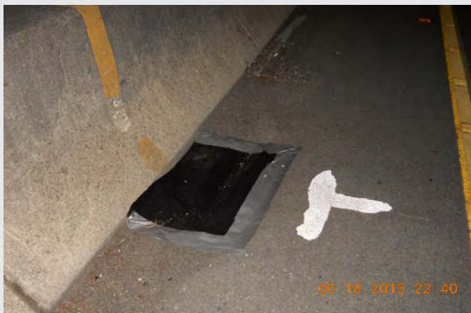
Figure 6. Photograph. Example of masking of drainage structures near HFST application.
