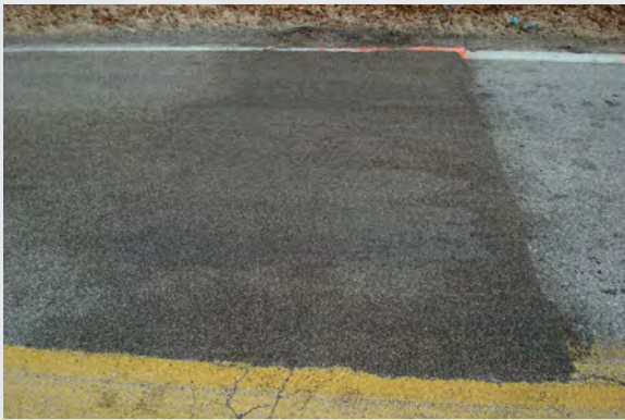
Figure 23. Photograph. Example of discoloration indicating uncured resin binder.
