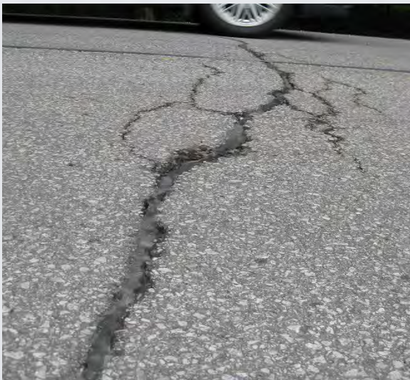
Figure 2. Photograph. Example of bituminous crack sealant in asphalt pavement.
