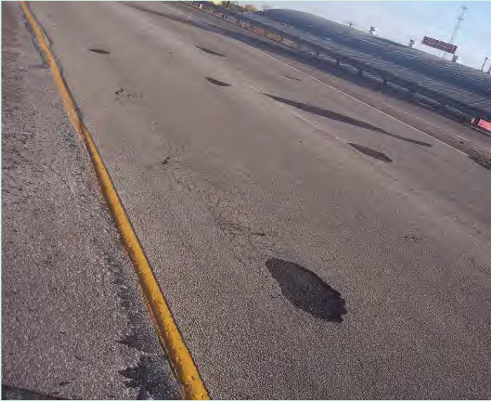
Figure 30. Photograph. Example of failure of underlying pavement leading to isolated failures (potholes) of HFST.
