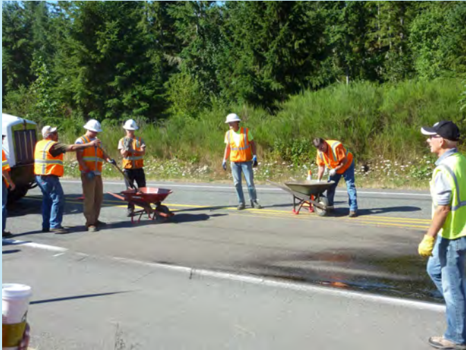
Figure 15. Photograph. Example of manual application of HFST aggregate.
