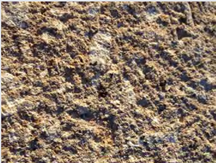
Figure 4. Photograph. Shotblast concrete surface with CSP = 5.
