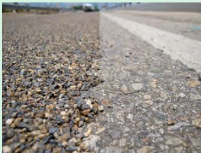
Figure 1. Photograph. HFST placed over a conventional asphalt pavement surface. 1
