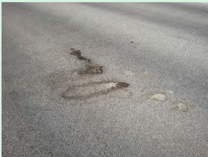
Figure 28. Photograph. Example of HFST discoloration likely caused by moisture.
