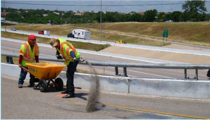
Figure 9. Photograph. Example of manual application of aggregate, broadcast by hand.
