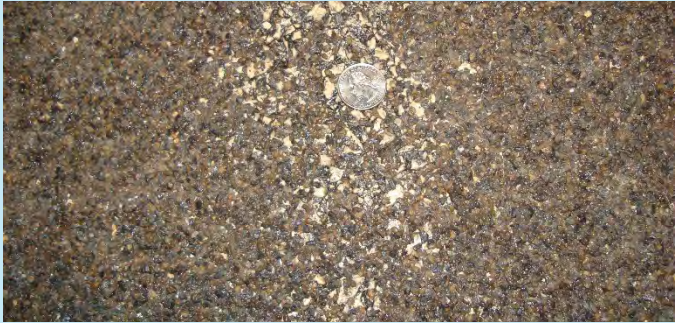
Figure 21. Photograph. Example of exposure of underlying pavement after sweeping.
