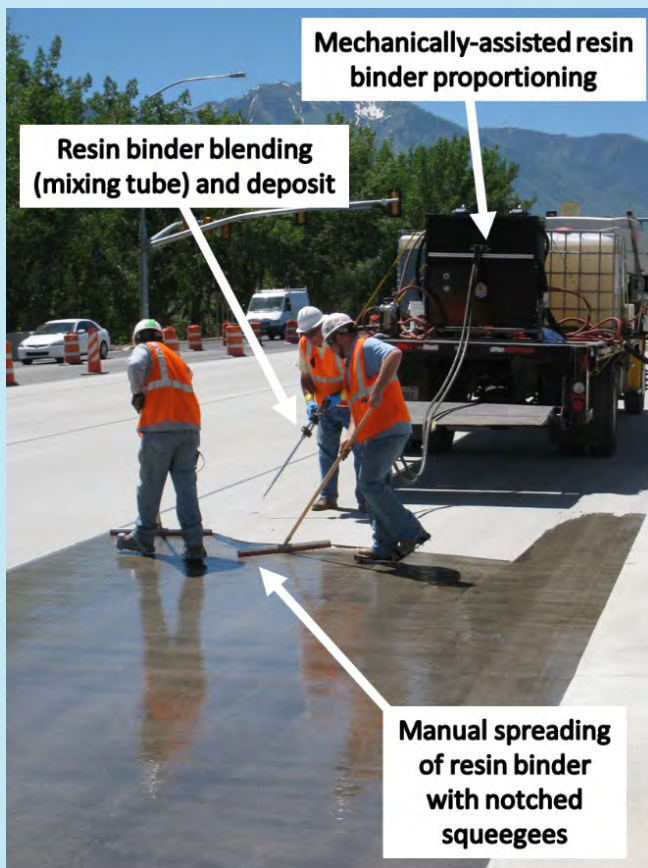
Figure 8. Photograph. Example of mechanically-assisted manual resin binder application.
