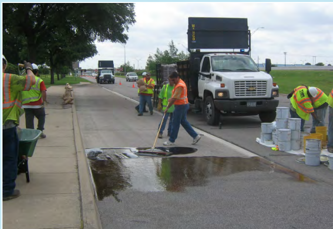
Figure 14. Photograph. Example of manual resin binder application.
