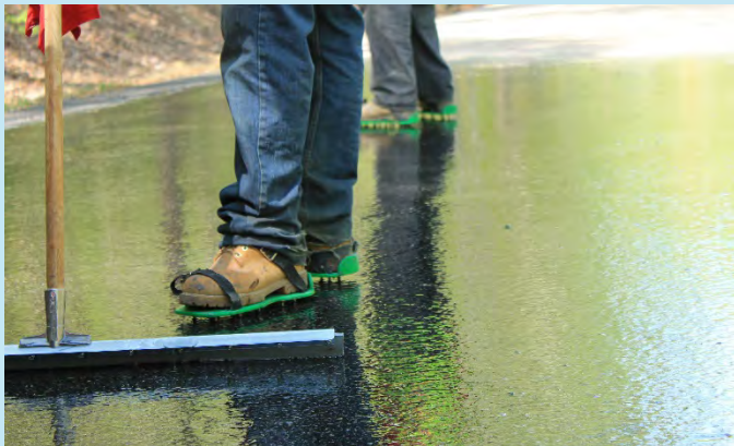
Figure 12. Photograph. Example of spiked shoes worn by squeegee operator.
