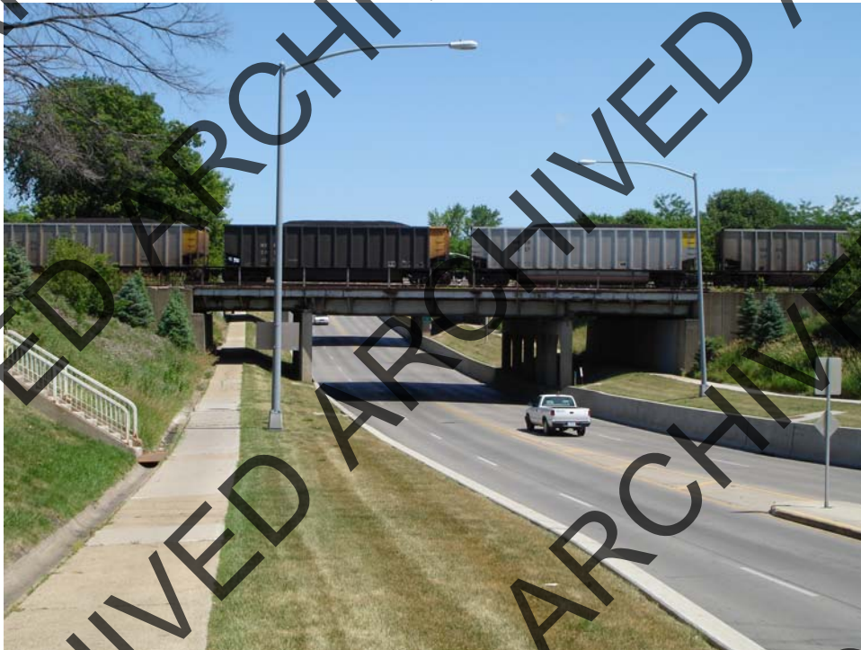
FIGURE 19 Sight distance at an undercrossing.
