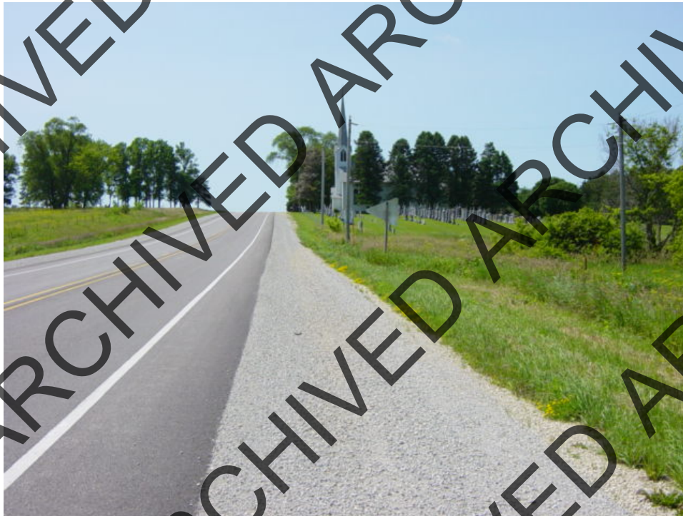
FIGURE 9 Pavement edge drop-off.
