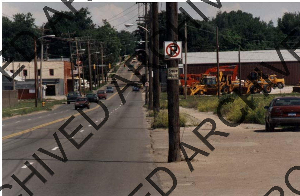
FIGURE 25 Lateral offset to obstruction is an operational offset and is not the same as clear zone.
