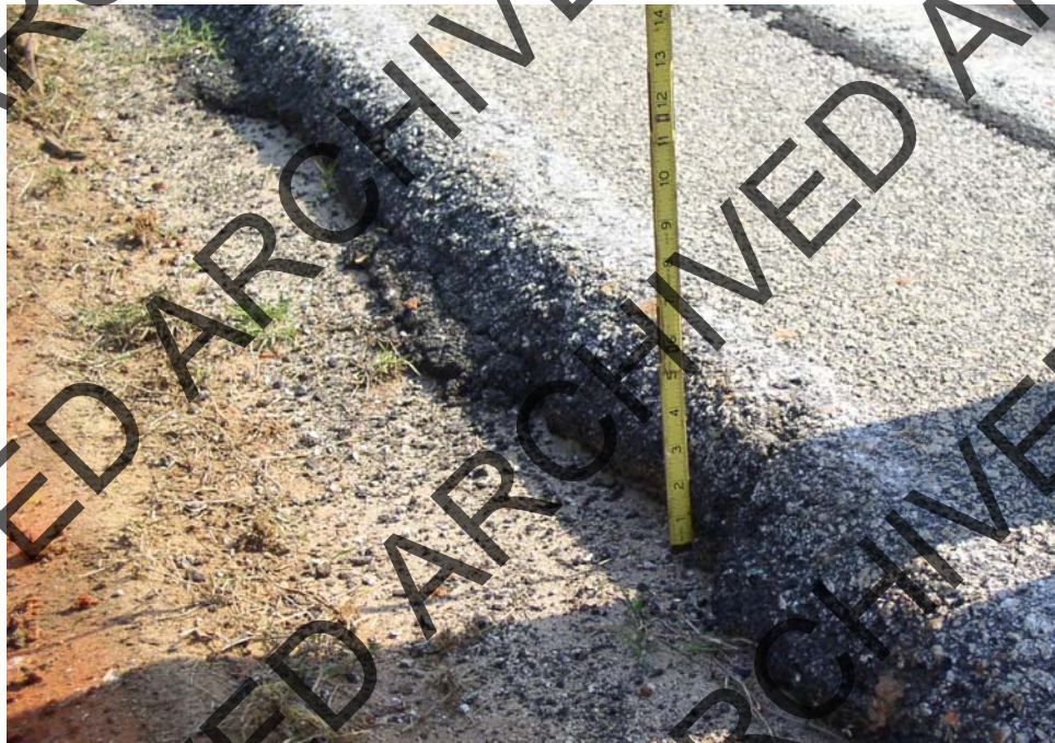
FIGURE 9 Pavement edge drop-off.
