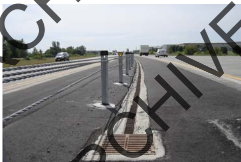
FIGURE 56 Continuous drainage system.
