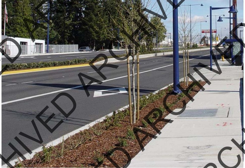
FIGURE 109 Sloped-down end section adjacent to turn lane.
