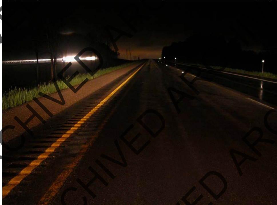
FIGURE 34 Painted edgeline rumble strips
