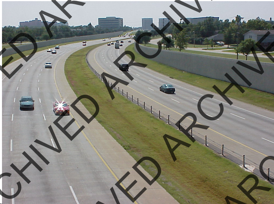
FIGURE 7 Shoulders on this urban freeway provide enough width for crash avoidance, storage of disabled vehicles, maintenance activities, and enforcement.
