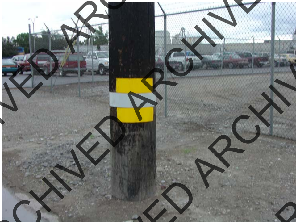
FIGURE 69 Reflective sheeting on utility poles.
