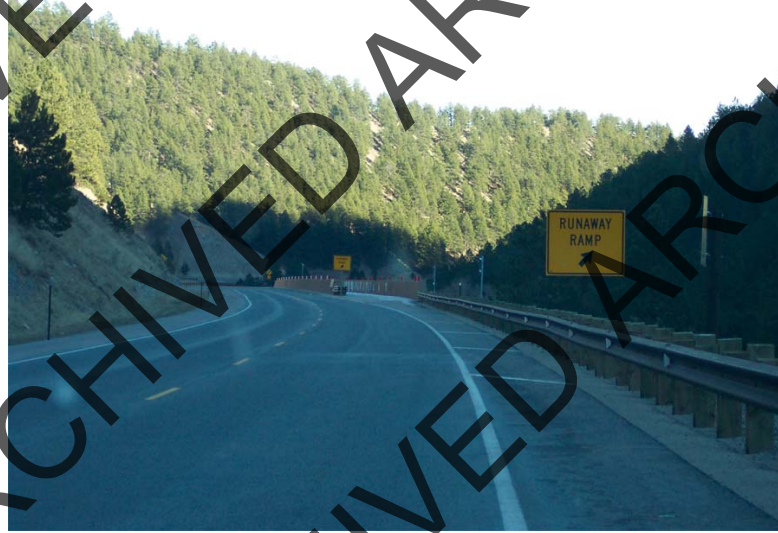
FIGURE 92 Runaway truck ramp A nearby ramp on the other side of the roadway was replaced because it required crossing the opposing lane of traffic.
