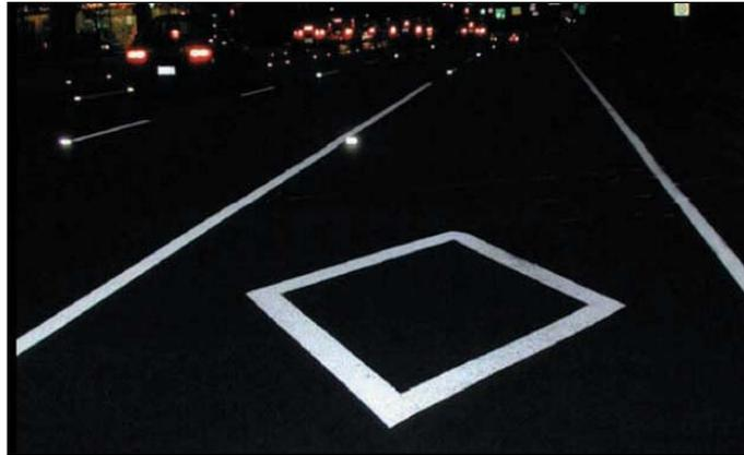
Figure 40 - Retro-Reflective Pavement Markings
