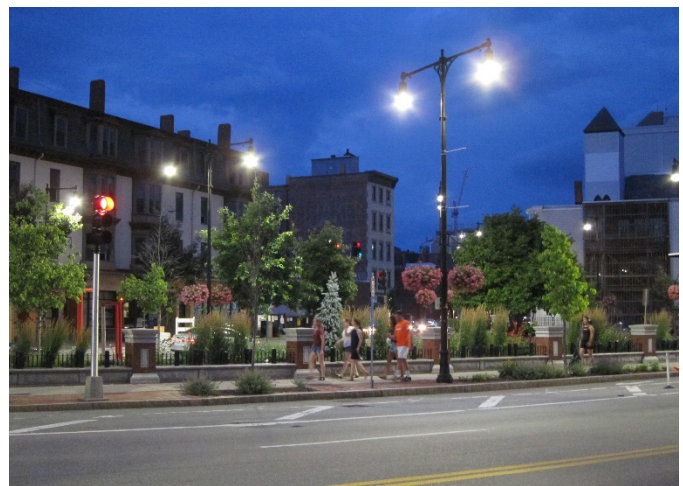
Figure 4. Roadway at night with street lighting. Source: WSP.
