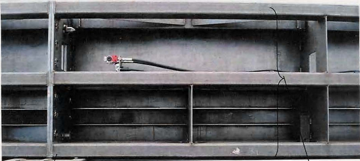
Top, mid, and lower beams with lower channel – 46” height (55-58” overall height w/ 9-12” clearance)
