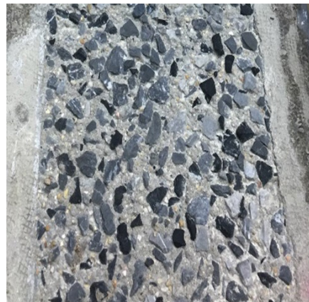
Figure 3. Photograph. Concrete substrate after hydromilling.
