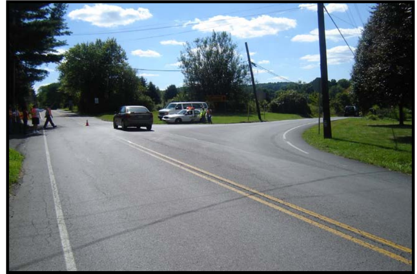
PA 412/PA 212 west intersection – looking northbound
