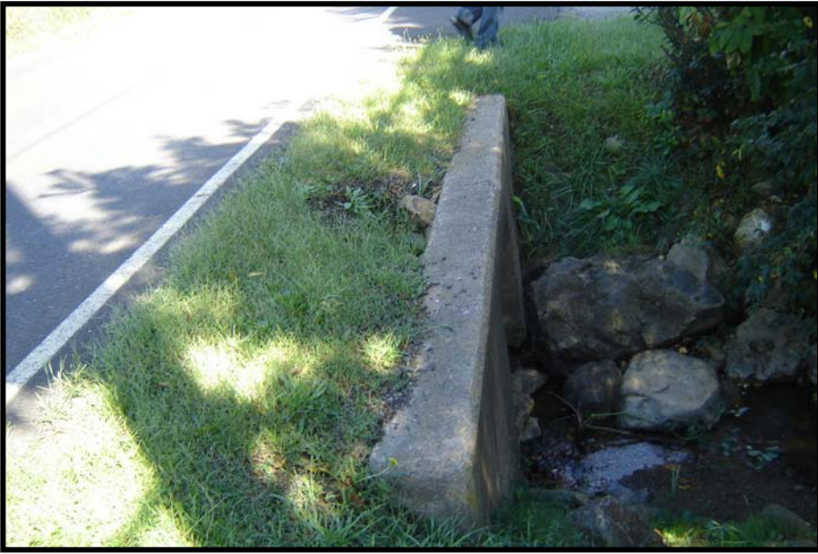
Culvert and headwall deterioration at 3398 Main Street.
