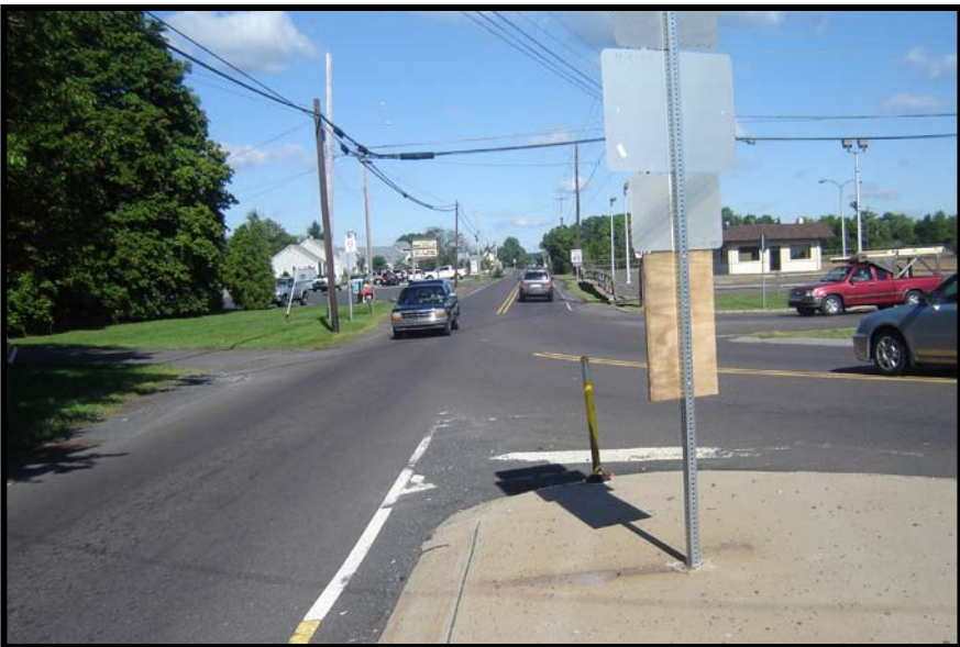
Faded pavement markings and illegal sign at PA 611/PA 412 intersection
