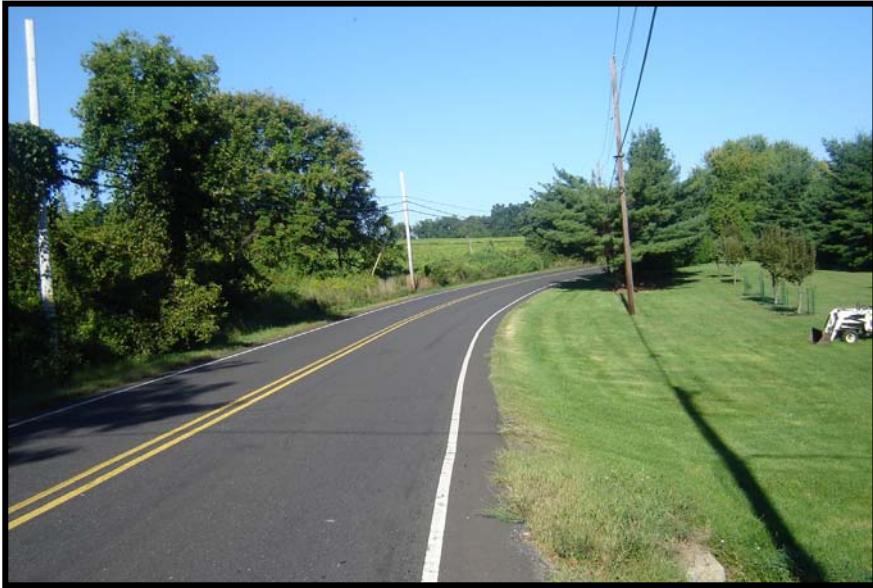
Downhill curve north of Bodder Road, no delineation
