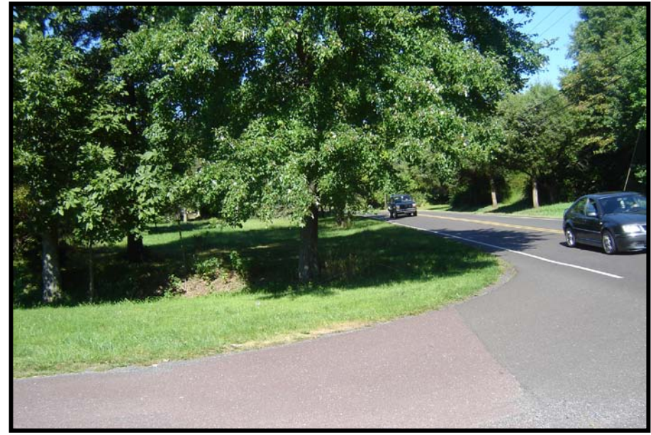
Meginnes Road approach to PA 412 – sight distance compromised by trees
