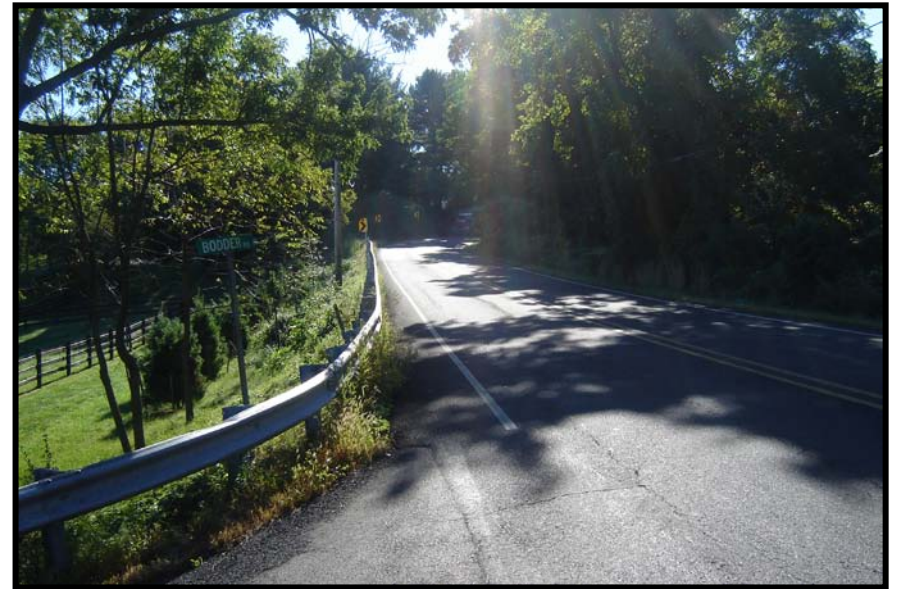
Bodder Road intersection looking southbound – curve warning signs
