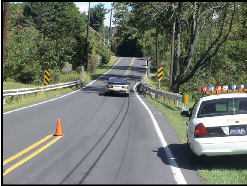
Southbound approach to the one lane bridge
