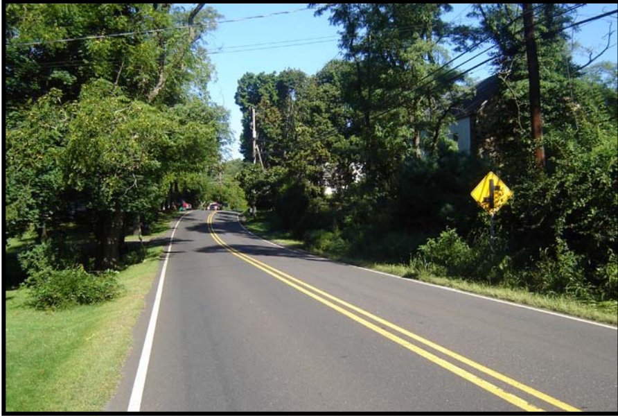
Intersection warning sign for Bursonville Road is blocked by trees
