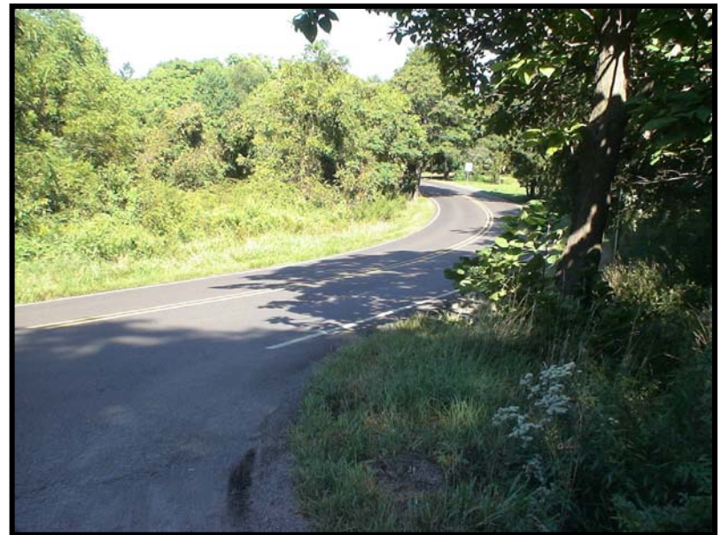
Buckwampum Road intersection looking north on PA 412
