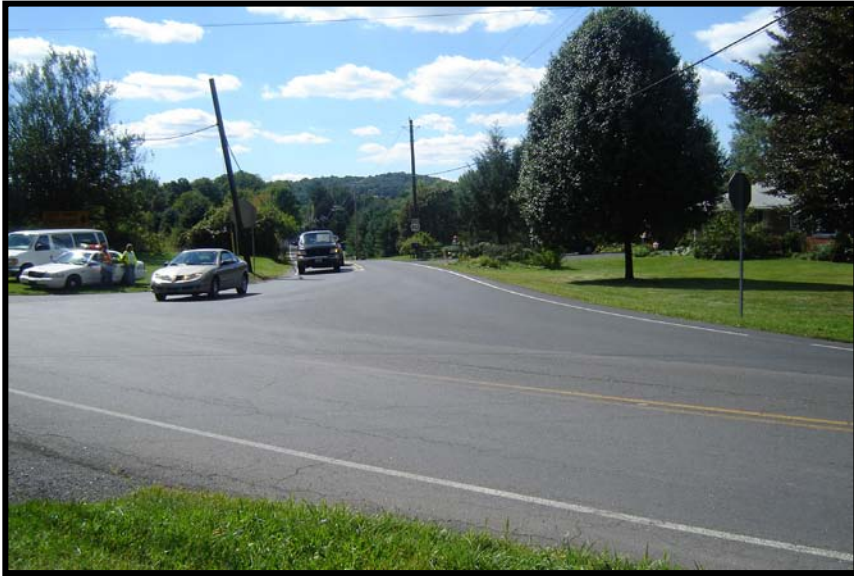
Skewed PA 412/PA 212 west intersection
