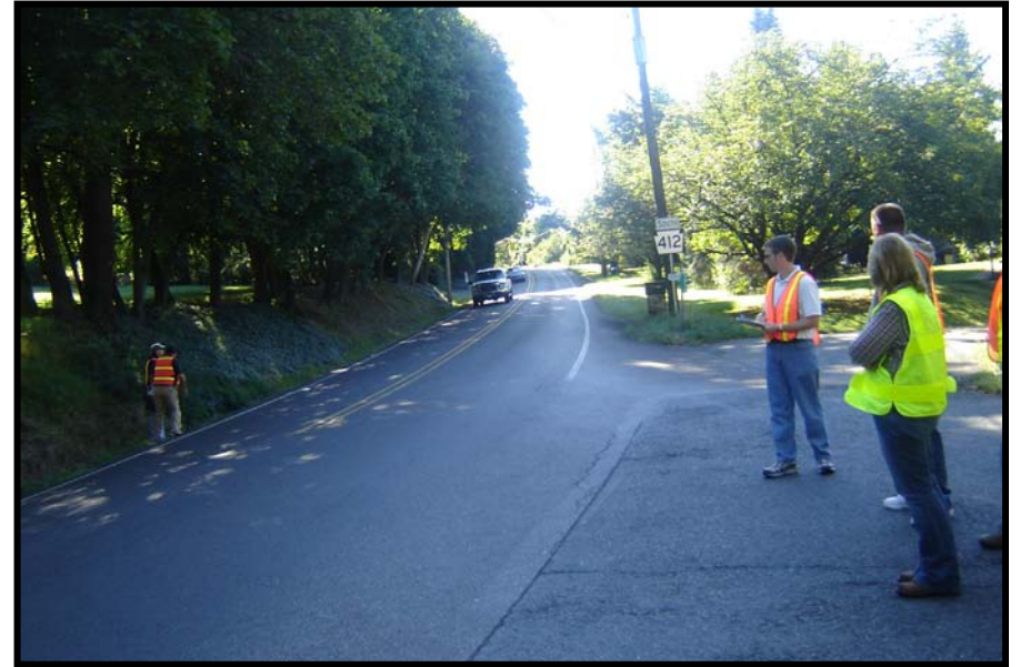
Slifer Valley Road intersection - Stopping sight distance to turn left on Slifer Valley Road is inadequate; excessive and inconsistent grades
