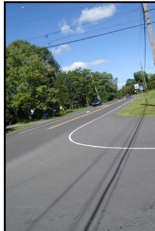
Gessner Road intersection evidence of vehicles leaving the roadway to make a right turn on to PA 412. Stop sign and markers are leaning.
