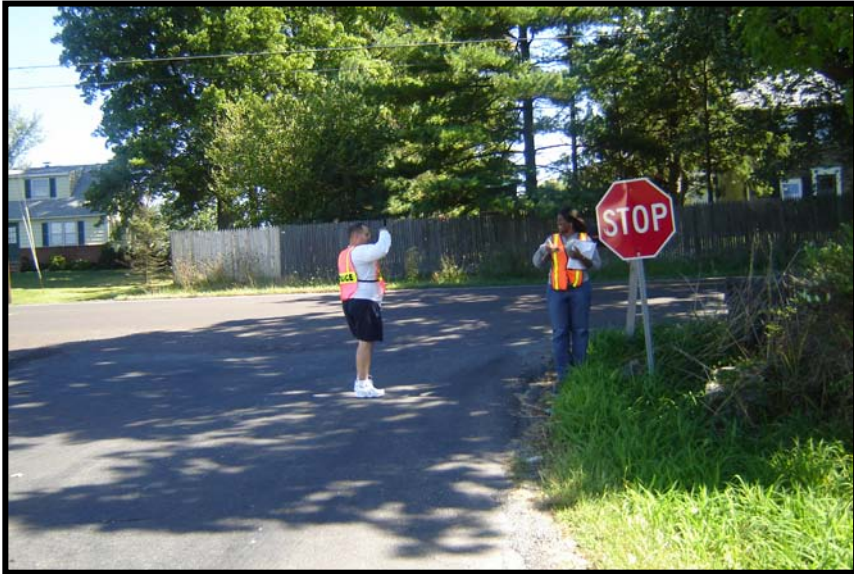
Stop sign at Park Drive West installed too low
