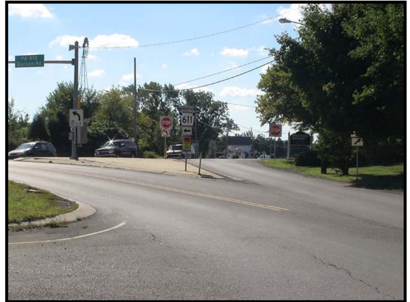
PA 611/PA 412 intersection looking eastbound
