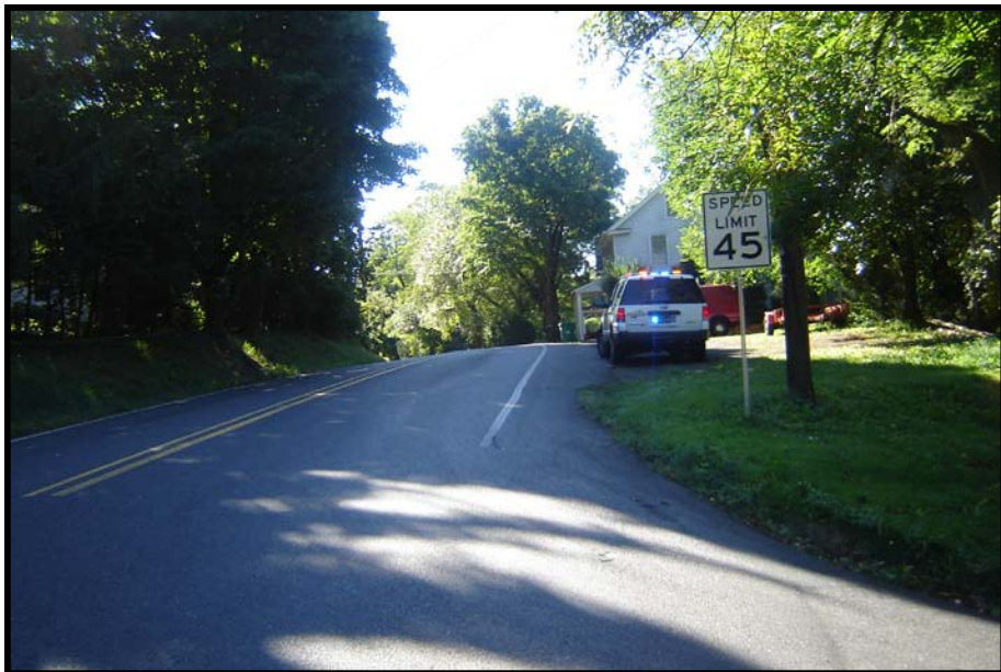
Sight distance at Bursonville Road is severely compromised due to PA 412 profile; 45 MPH speed limit sign at the curve
