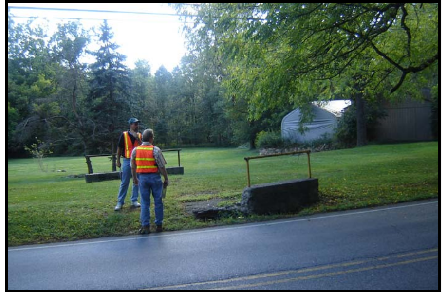
Old bridge wall across from Funks Mill Road is in the clear zone
