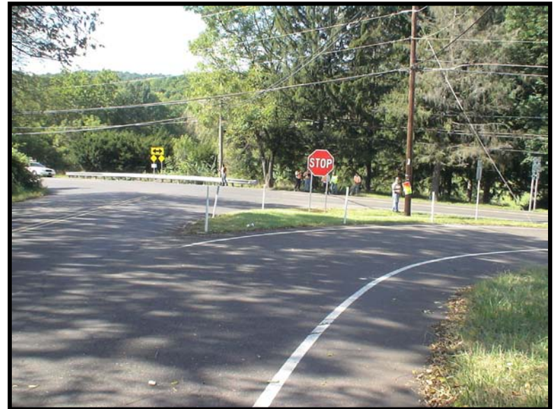
Northbound approach of PA 412/PA 212 east intersection
