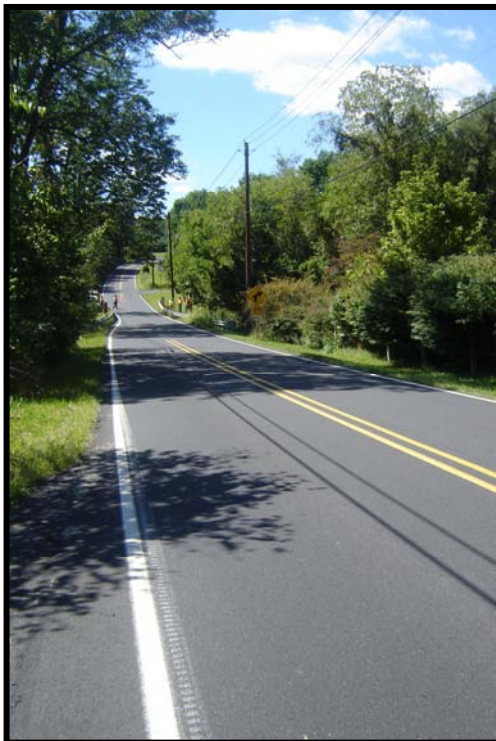
Northbound approach to the one lane bridge
