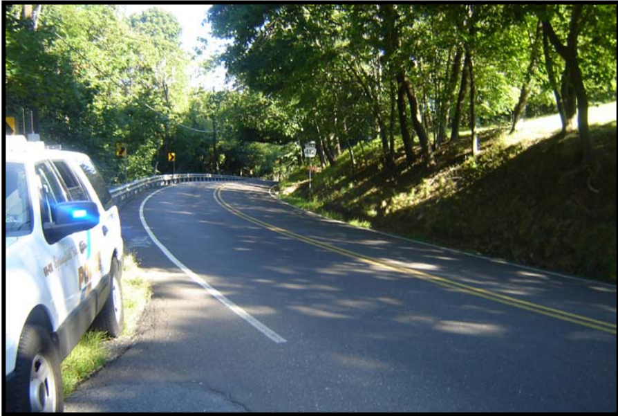
At Slifer Valley Road PA 412 is covered by tree canopy. Excessive and inconsistent grades.
