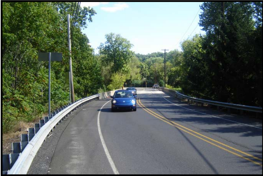
Bridge north of Cooks Creek Road
