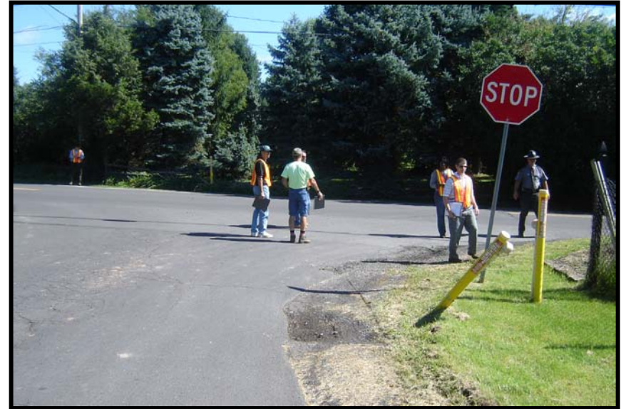
Gessner Road intersection evidence of vehicles leaving the roadway to make a right turn on to PA 412. Stop sign and markers are leaning.
