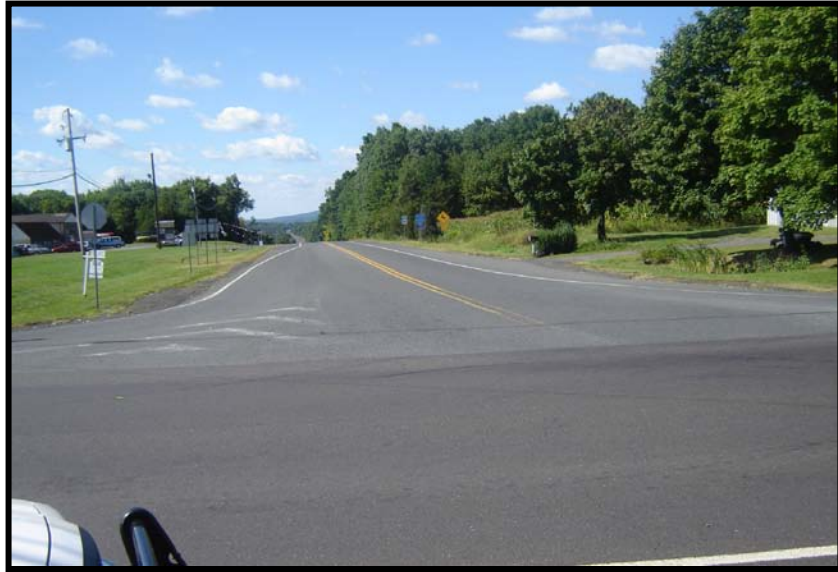
Wide intersection approach at Mountain View Drive
