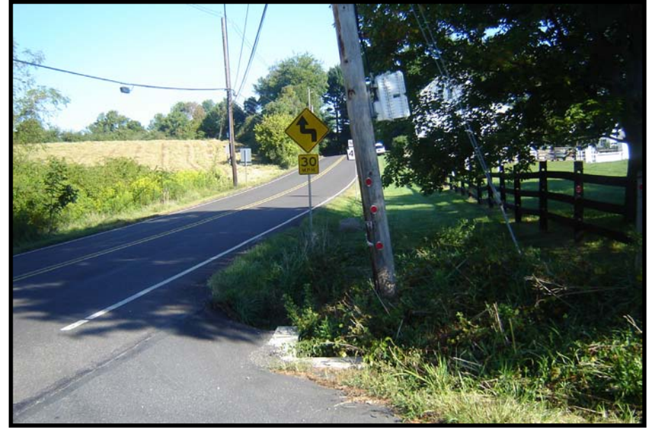
Signs and utility pole at Lehnenberg Road compromise sight distance
