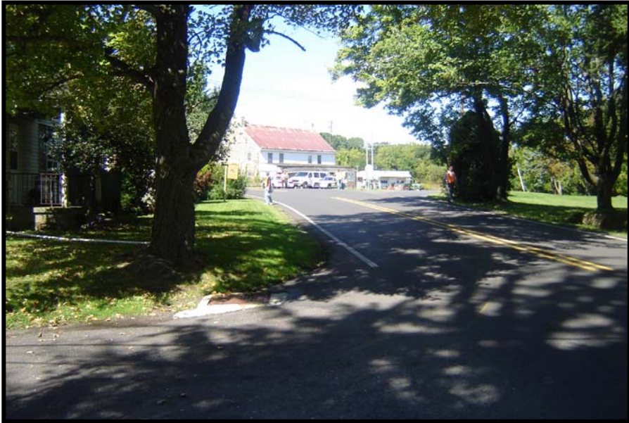
Stony Garden Road looking northbound on PA 412, sight distance compromised – curve and bushes
