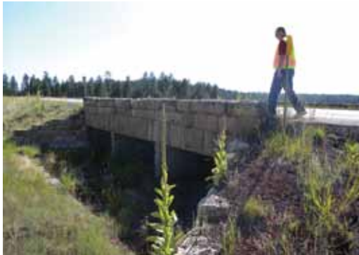
RSAs EXAMINE ROADWAY AND ROADSIDE FEATURES THAT MAY POSE POTENTIAL SAFETY ISSUES.
