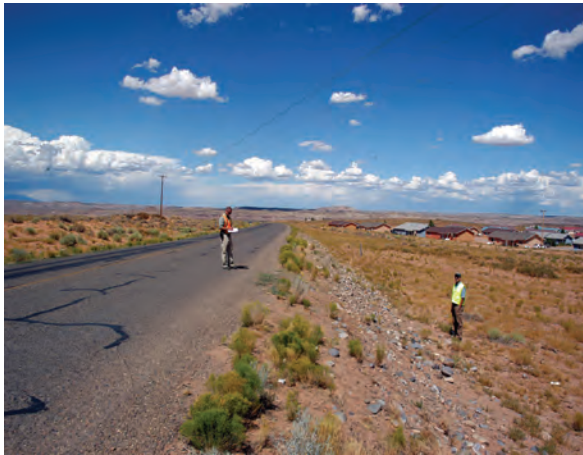
N-35 IN RED MESA, UTAH. PHOTO SHOWS LIMITED PAVEMENT WIDTH, LACK OF DELINEATION, AND CLOSE PROXIMITY OF ROADSIDE HAZARDS.
