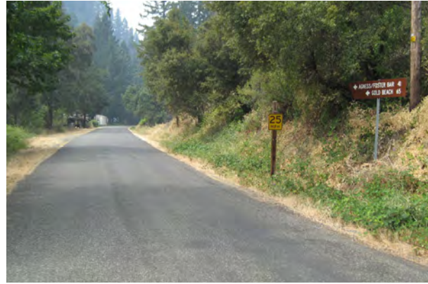
BLM SEGMENT (BLM ROAD 34-8-36), NEAR THE INTERSECTION WITH PEAVINE/SERPENTINE SPRINGS ROAD. A SPEED LIMIT SIGN (25 MPH) IS POSTED AT RIGHT. THE UNMARKED PAVEMENT CAN ACCOMMODATE TWO LANES OF TRAFFIC.
