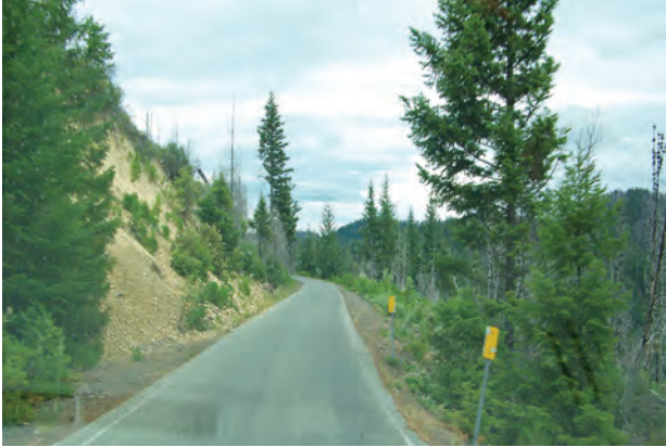
FS SEGMENT (FS ROAD 23), SHOWING A SINGLE-LANE WITH NO TURNOUTS. FOG LINES ARE VISIBLE ON BOTH SIDES OF THE PAVEMENT, ALONG WITH REFLECTIVE DELINEATORS AT RIGHT.
