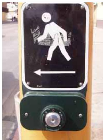
**Figure 23. Call Buttons Tested in Miami**
