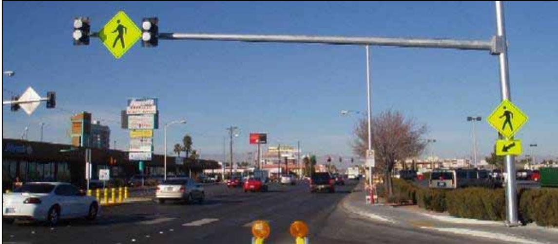
**Figure 25. Overhead Flashing Beacons Tested in Las Vegas**
