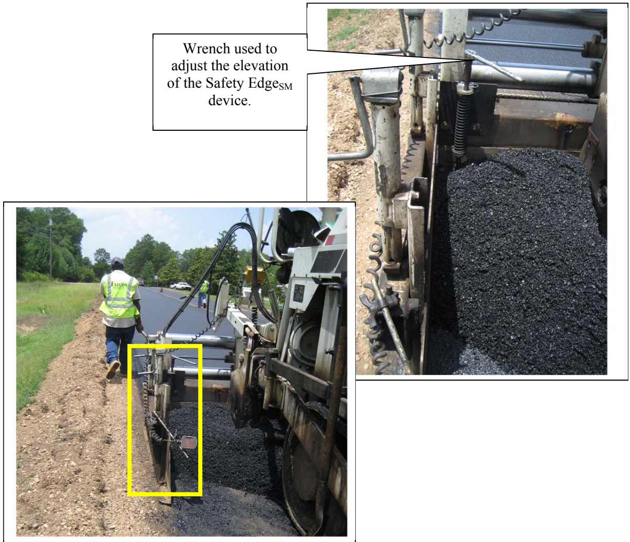
Figure 12. Safety Edge SM adjustment for raising and lowering the device.
