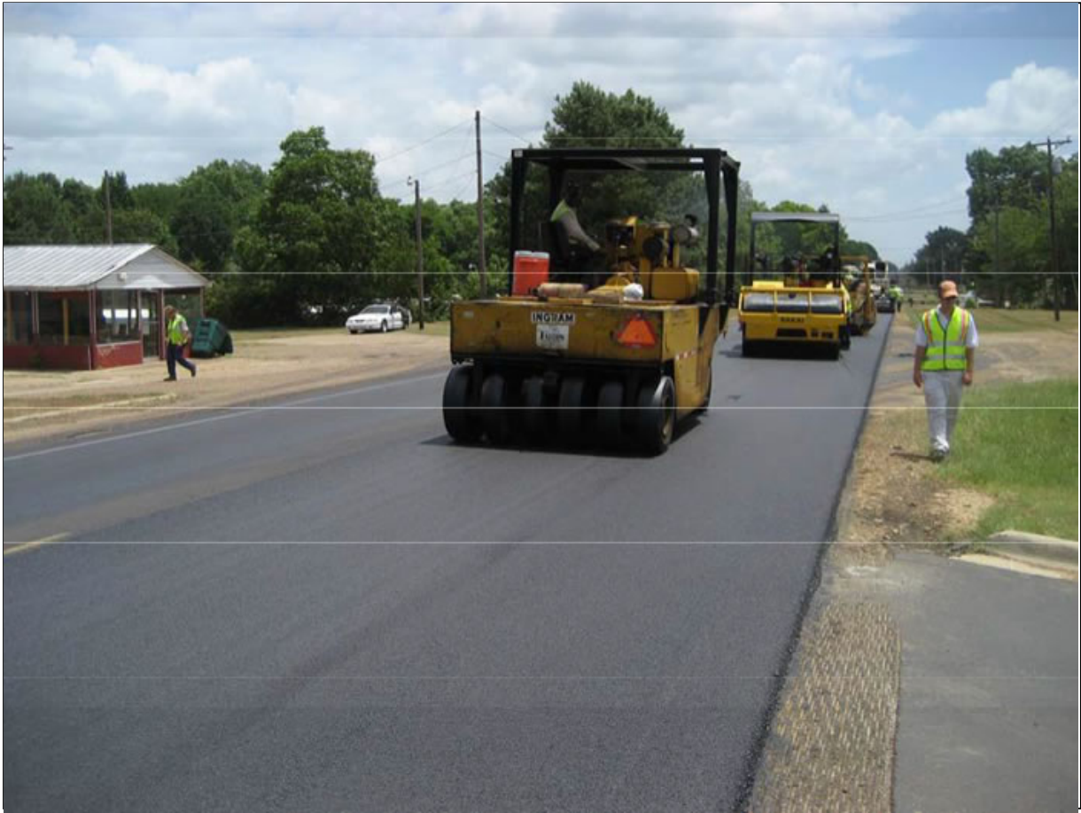
Figure 13. Rolling the Safety Edges SM with standard rollers – No special rollers are required.
