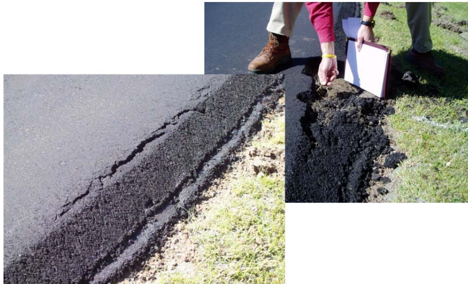
Figure 11. Longitudinal crack due to Safety Edge SM break point located on unimproved shoulder.
