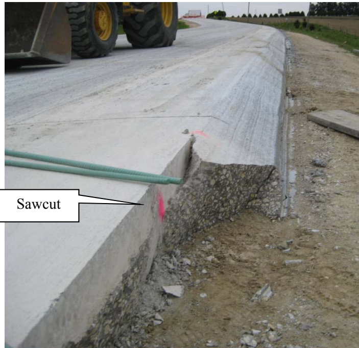
Figure 4. Sawcut on a PCC project at an intersection to remove the Safety Edge SM .
