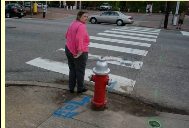
Photo shows where a hydrant is located in the middle of the curb ramp, obstructing access between the sidewalk and crosswalk.
