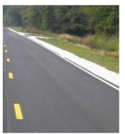
As with conventional paving, the shoulder material is brought flush with the top of the pavement before the project is considered complete. Again, drivers are not initially exposed to a drop-off.
