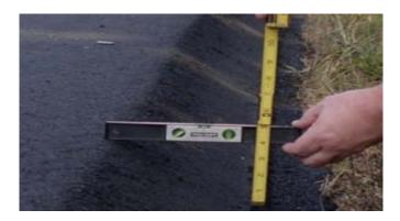
There is one change with the Safety Edge—a shoe is attached to the paver to consolidate the edge material into a tight 30-degree shape as it comes off the screed. Compactive rolling of the rest of the pavement proceeds normally, as no additional compaction is necessary.
