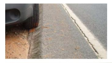
(if a proper shoe provided the intended compaction at laydown), so there is no lost material in the process. More importantly, the 30-degree edge that is exposed does not induce tire scrubbing. Drivers who have dropped a tire over this edge are very likely to be able to return to their lane without losing control as they attempt to steer back onto the pavement.
