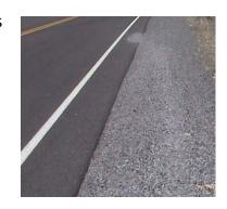
After a few months, the shoulder begins to settle and the edge is exposed. Erosion also works on this material to wash it away. On narrow pavements, or in certain locations like curves or mailboxes, the unpaved shoulder
