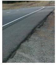
may be worn down by tires as well. The loose asphalt at the edge is lost with the shoulder material and the hard pavement edge is nearly vertical, with a rounded top. This edge can cause tire-scrubbing in a roadway departure.
