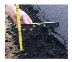
In the conventional asphalt paving process, approximately 80 percent of compaction is achieved by the screed, then a series of rollers
