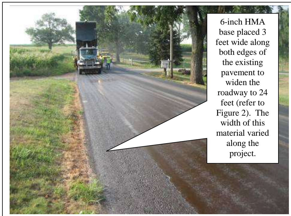
Figure 4. Additional HMA base material placed along each edge of the roadway.
