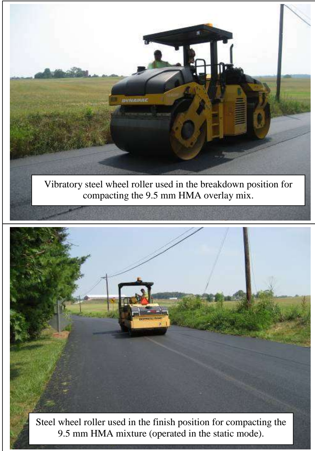
Figure 21. Two steel wheel rollers used to compact the 9.5 mm HMA mix.
