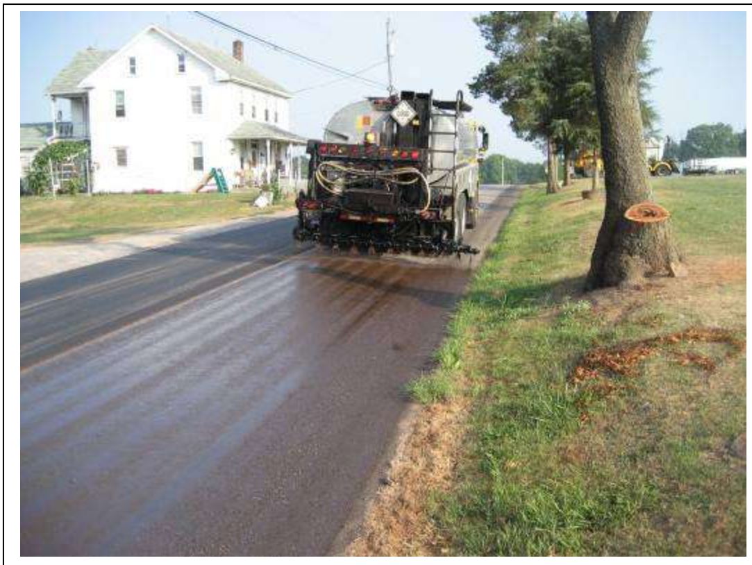
Figure 15. An emulsion was used as a tack coat prior to HMA placement (note the material that was added to the edge of the pavement to widen the roadway).
