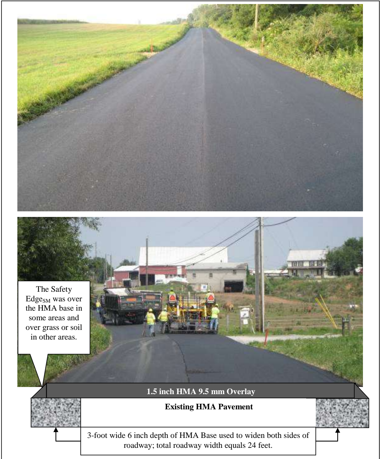
Figure 2. General overview of the 1.5 inch HMA layer placed along the project and pavement cross section provided by the Pennsylvania DOT.
