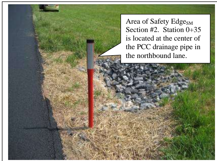
Figure 7. Reference marker for Safety Edge SM Section #2.
