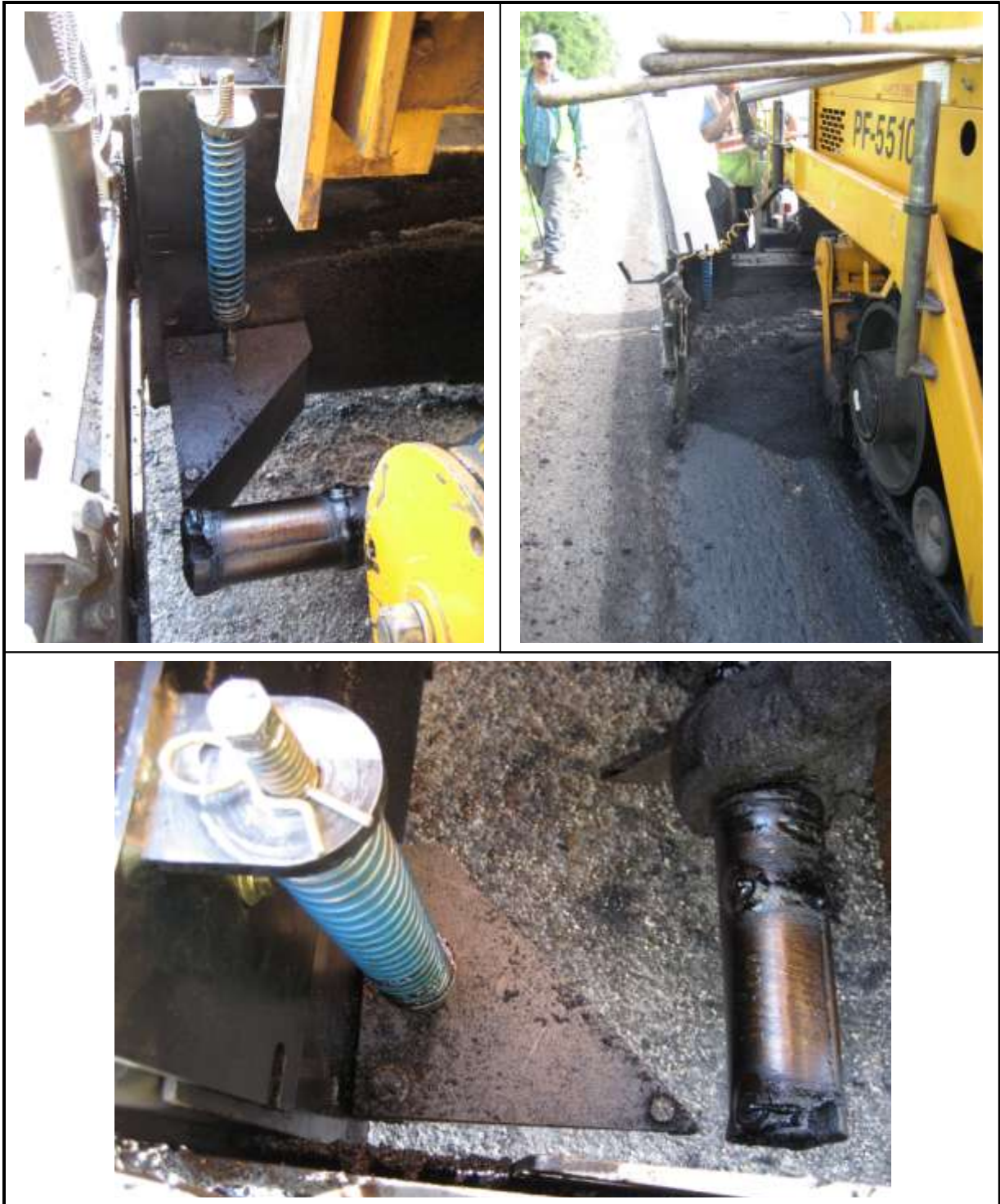
Figure 15. TransTech Shoulder Wedge Maker device attached to the screed.
