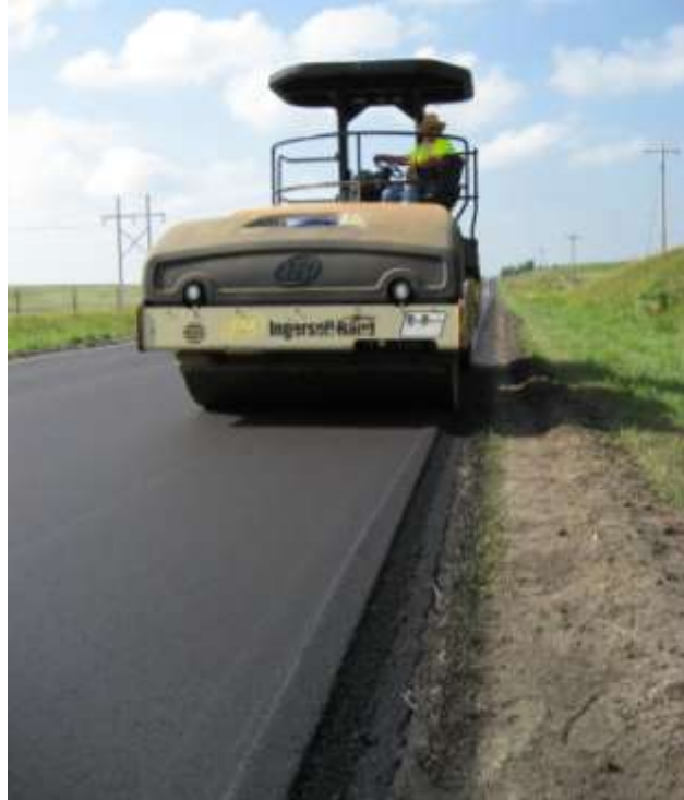
Figure 21. First pass of the Ingersoll-Rand finish roller along the Safety Edge SM .
