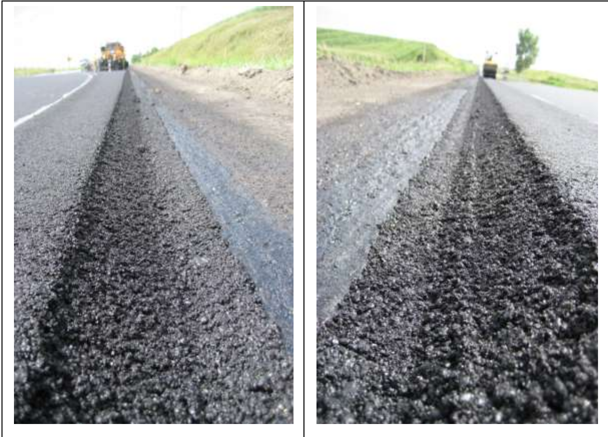
Figure 16. Typical surface texture and slope of the Safety Edge SM sections.
