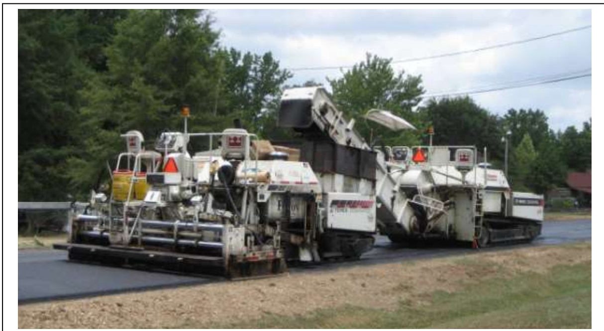
Figure 15. Equipment used to place the HMA overlay.
