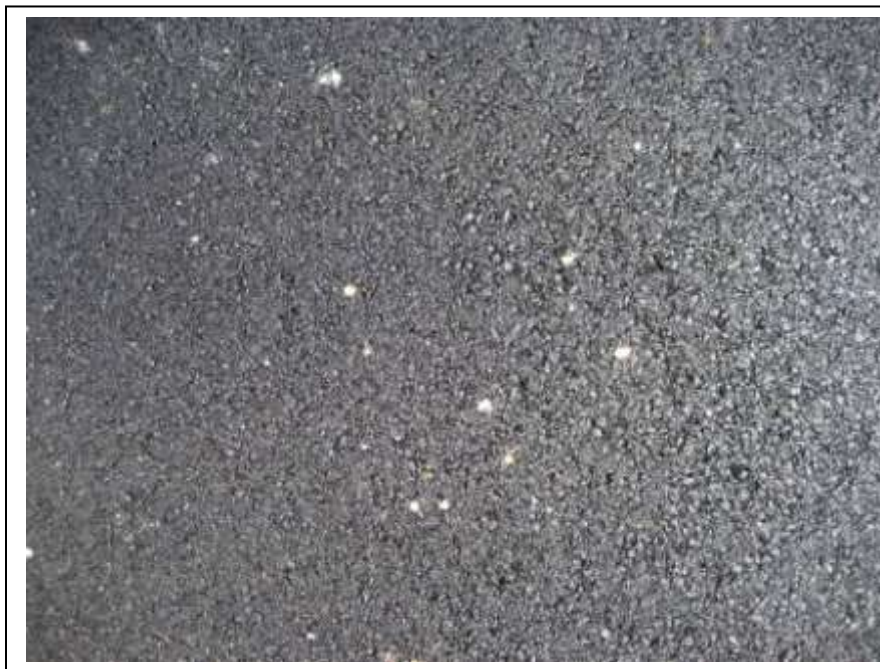
Figure 21. Surface texture of the 9.5 mm HMA overlay after final rolling.
