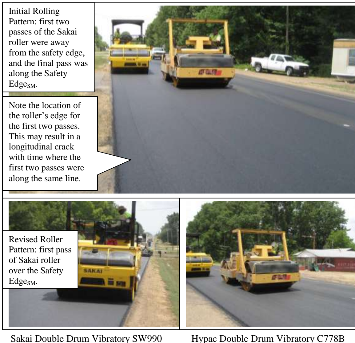
Figure 18. Two double drum vibratory steel wheel rollers were used in parallel in the breakdown position to compact the 9.5 mm HMA mix.
