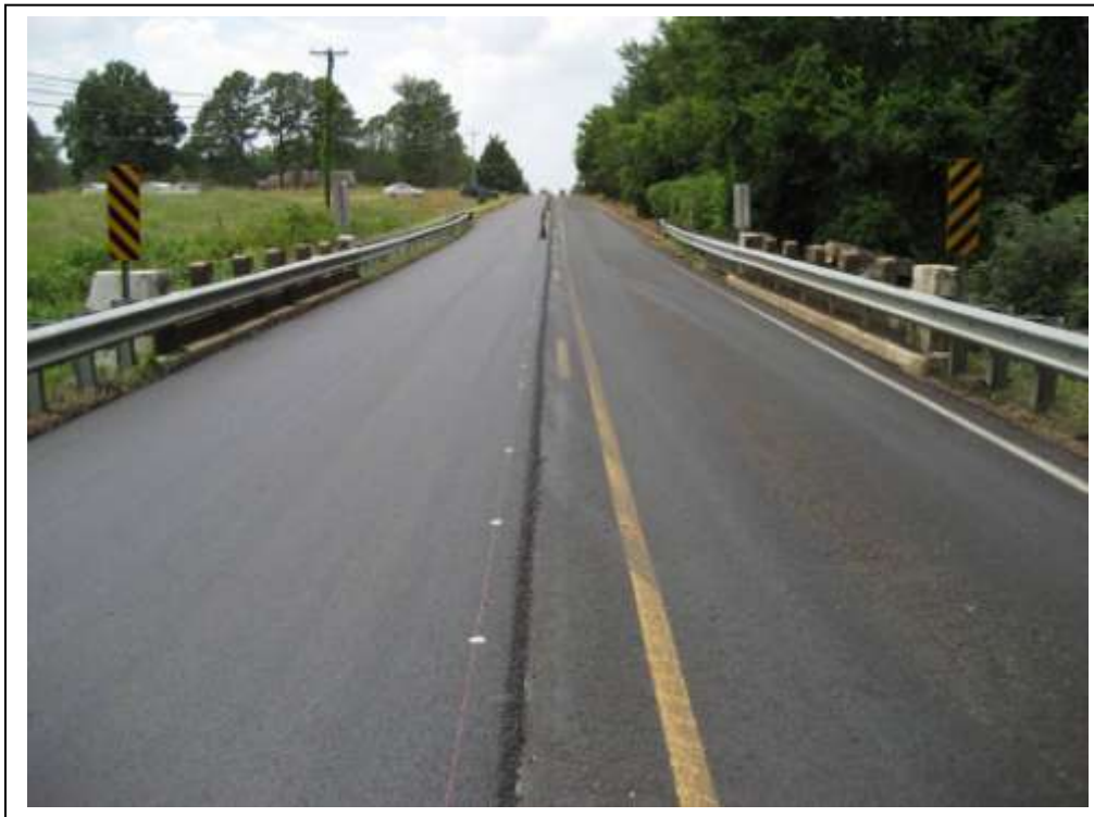
Figure 23. One of the narrow bridges located on the project (about 22-feet wide).
