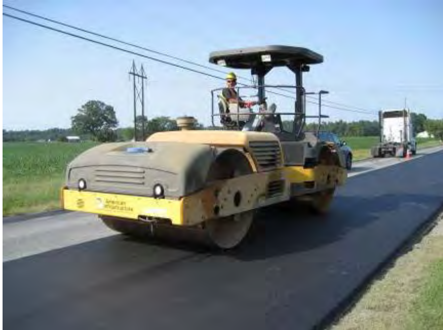
Figure 19. Rollers used for compacting the 9.5 mm WMA overlay mixture.
