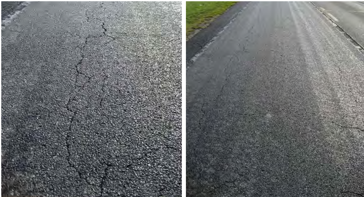
Figure 2. Typical condition of the existing surface (with tack coat applied).
