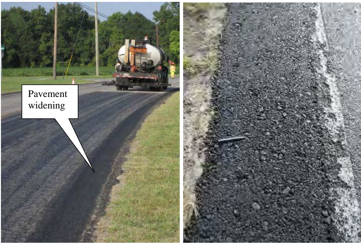
Figure 5. 1.0-ft widening strip placed on both sides of the roadway.
