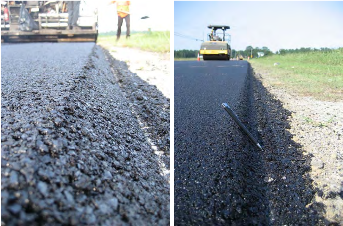
Figure 17. Typical surface texture and slope of the Safety Edge SM sections.
