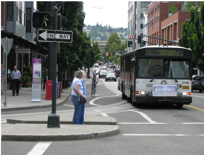
Pedestrian crossings at intersections can be enhanced by adding islands to help break the crossing into shorter distances while providing additional protection and improving visibility for all road users. Credit: Laura Sandt, PBIC Image Library.
