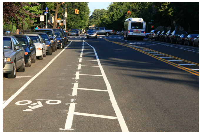
Buffered bike lanes provide additional separation from motor vehicle traffic and can enhance comfort and safety for bicyclists as a result. Credit: Steven Faust, PBIC Image Library.
