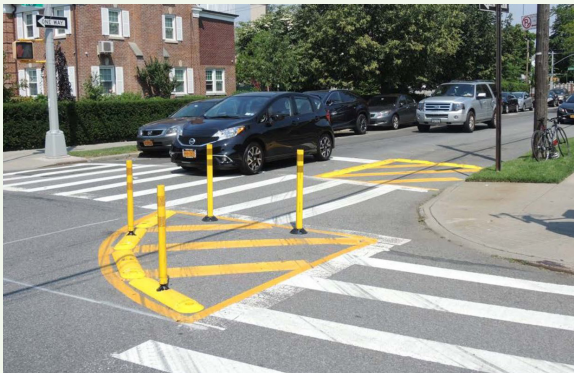
Low-cost treatments to tighten corners, as shown above, allowed NYCDOT to treat many of the locations where left turning conflicts were identified. Credit: NYC Vision Zero Year Three Report. https://www1.nyc.gov/assets/visionzero/downloads/pdf/vision-zero-year-3-report.pdf
