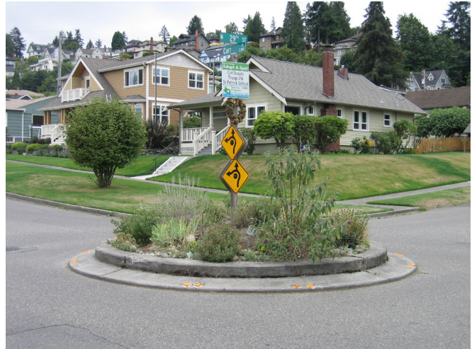
Neighborhood traffic circles can be used in residential areas to reduce the need for signals or all-way stops while also controlling speeds. Credit: Carl Sundstrom, PBIC Image Library.
