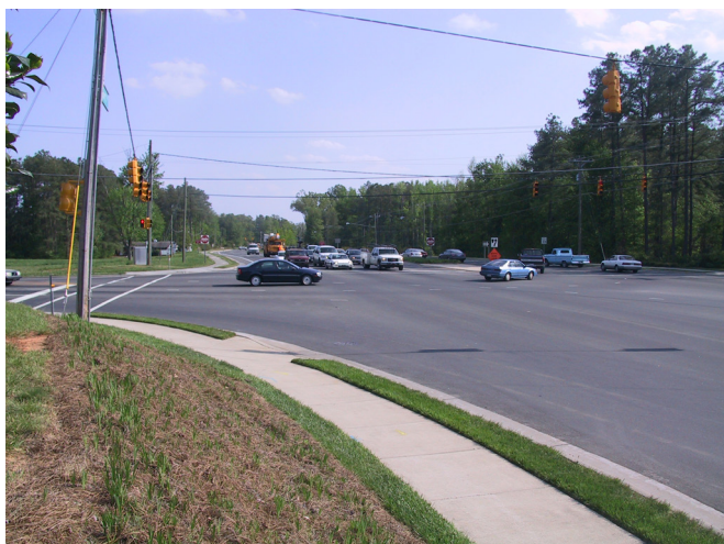
Designing intersections to accommodate turns by large vehicles may result in corners that facilitate faster turning vehicle speeds, as well as longer crossing distances. Credit: Libby Thomas, PBIC Image Library.
