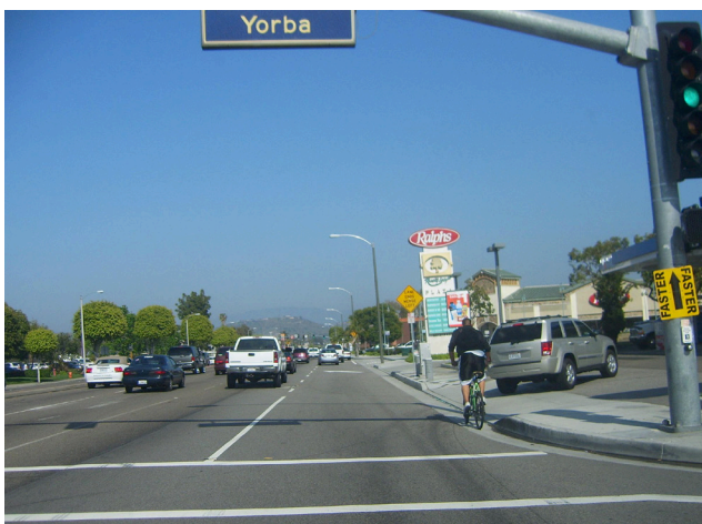
Multilane roads developed to prioritize automobiles often lack appropriate bicycle facilities. As speeds and volumes increase, a simple shared lane does not provide bicyclists with a comfortable, safe option. Credit: Nicole Schneider, PBIC Image Library.
