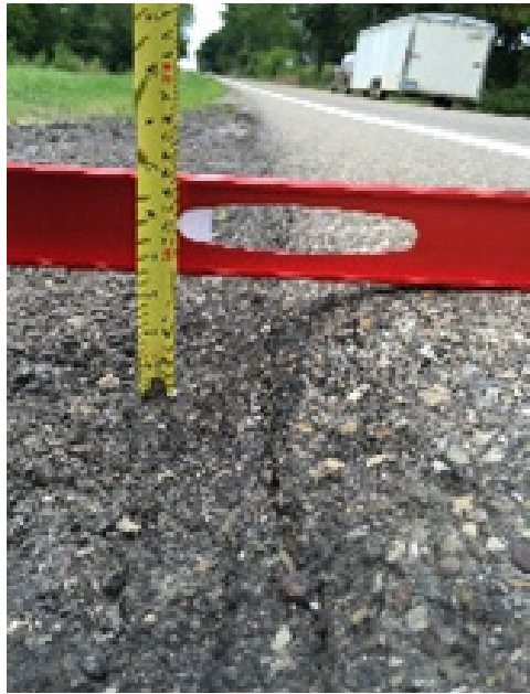
Figure 8. Photo. Example of Ohio SafetyEdge SM Treatment Site (Coshocton County, State Route 83, Curve to the Right).
