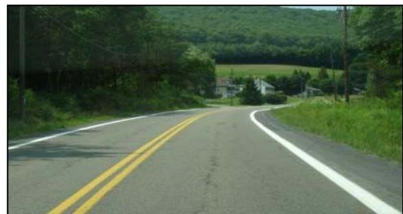
*Figure 11. Photo. Roadway with 8-inch edge line.*
