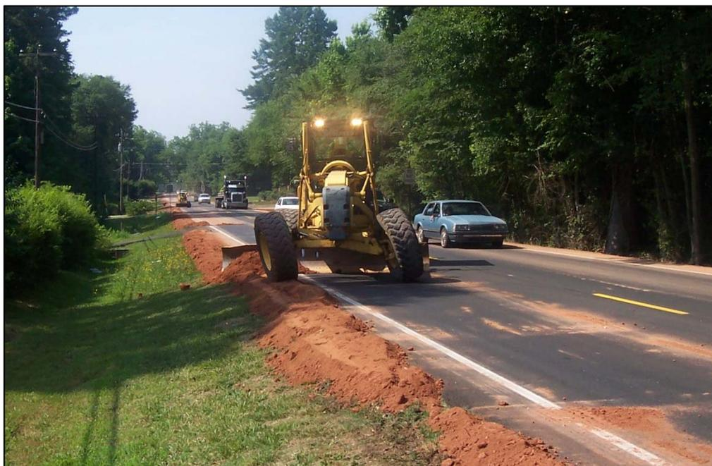
**Figure 46. Photo. Backfilling against newly installed Safety Edge<sup>SM</sup>.**
