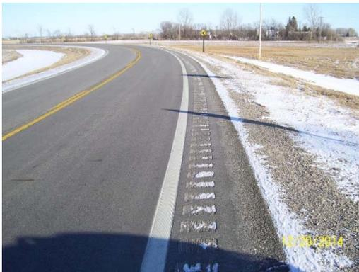
**Figure 6. Photo. Adding narrow paved shoulders (2 feet) to existing top width. Includes rumble strips and Safety Edge<sup>SM</sup>. Source: MnDOT.**
