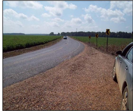
**Figure 68. Photo. Intersection with aggregate scattered on paved roadway.**
