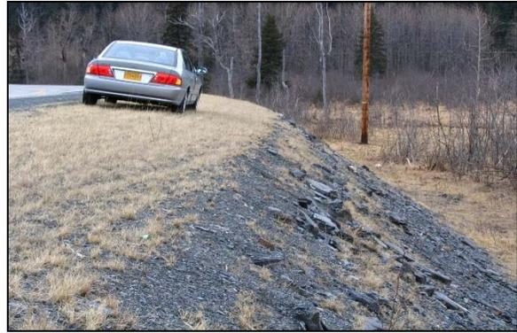
**Figure 51. Photo. Typical barnroof slope design.**
