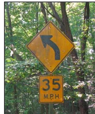
Figure 38. Photo. Low Retroreflectivity sign example.
