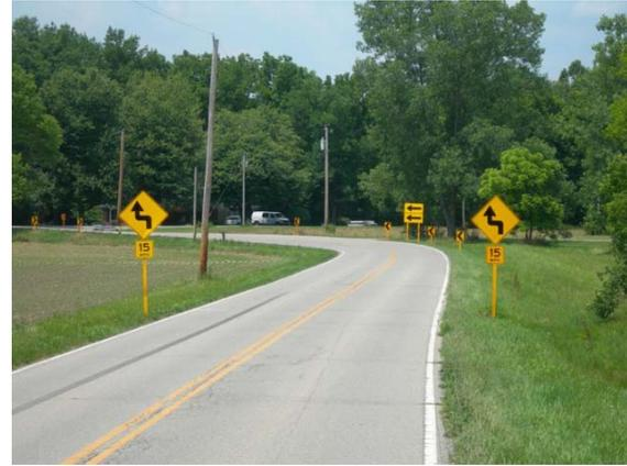
*Figure D-2. Photo. A curve on a rural, two-lane road after signage updates through the Horizontal Curve Program.*
