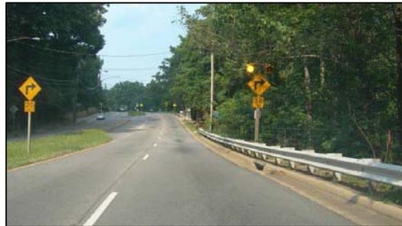
*Figure 29. Photo. Doubling-up of the sign was used at this site because tree limbs partially blocked the right side sign.*
