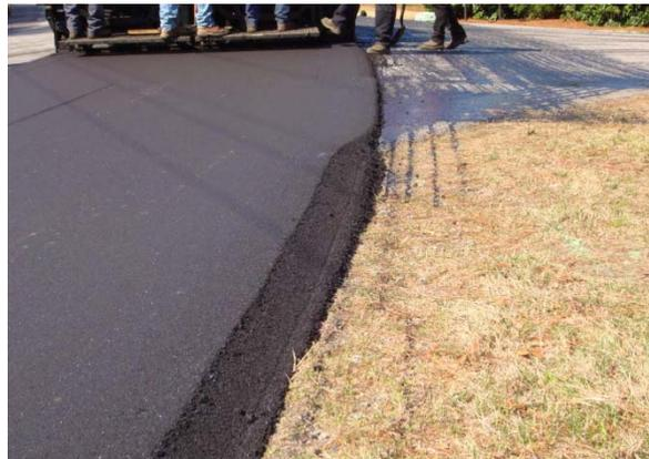
**Figure 45. Photo. Pavement with and without the Safety Edge<sup>SM</sup>.**
