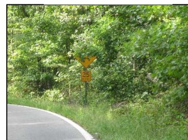
Figure 39. Photo. Curve warning sign covered by foliage.
