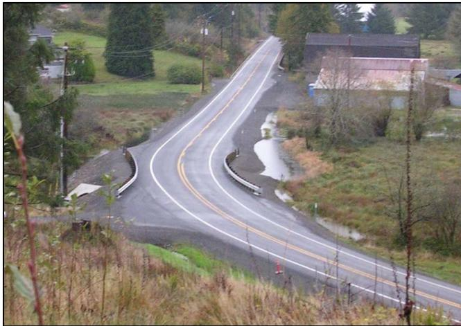
**Figure 67. Photo. Intersection with paved approach.**
