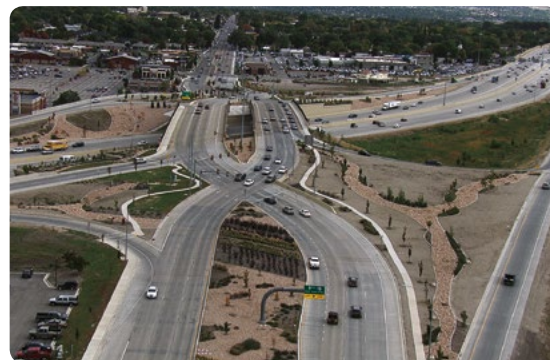
View of the Pioneer Crossing DDI Source: DDI Case Study Video FHWA-SA-14-043
