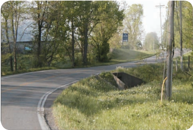
South Market Street before improvements
