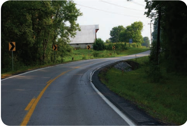
South Market Street after improvements
