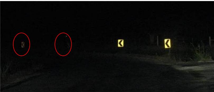
***When signs are out of proper alignment, they will not be as visible at night.***
