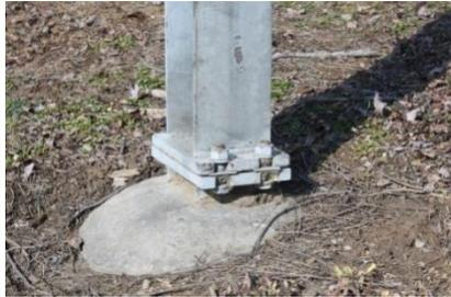
***I-beam steel posts with a slip base are needed for larger roadside guide signs.***
