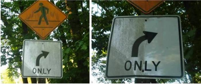
***Signs under a tree canopy are often covered with mold (left photo) which can easily be cleaned (right photo, right half of sign).***
