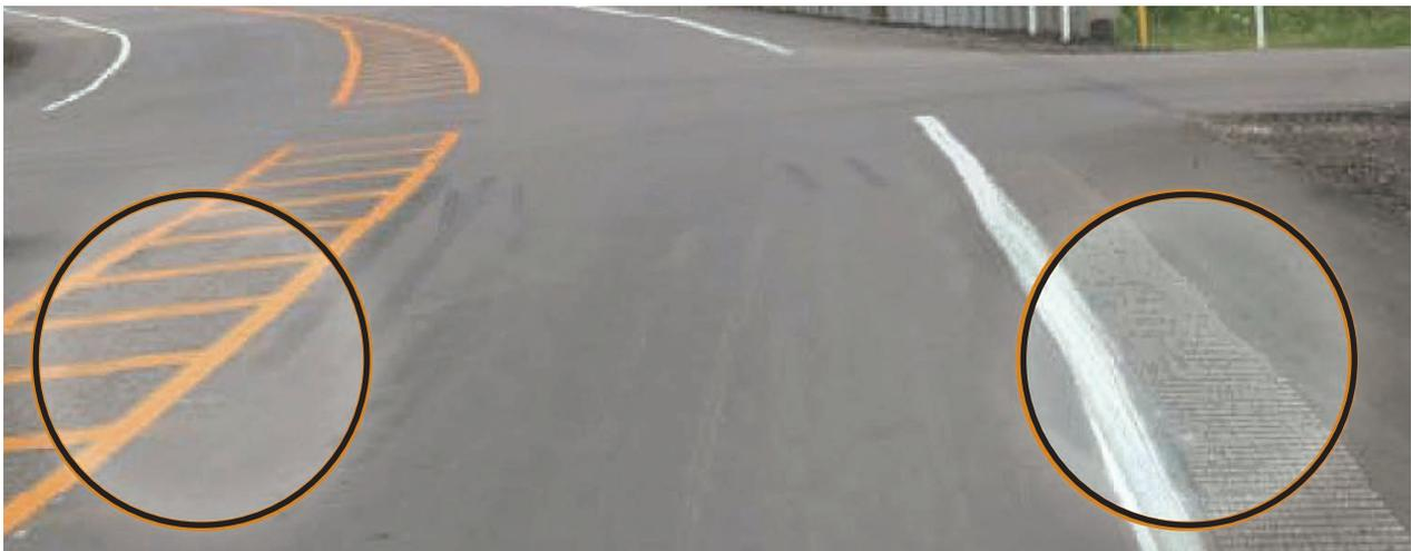
Figure 6: Lane Narrowing Using Rumble Strips
