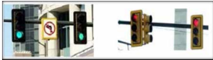
Figure 3. Signal Backplates with No Reflective Strip (left) and Signal Backplates with Yellow Retroreflective Strip (right)
