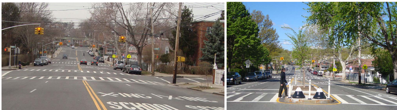
Figure 19. Allerton Ave, Bronx, New York City: Road Diet with Left Turn Bays, Pedestrian Refuge Islands and Bike Lanes (installed 2009)
