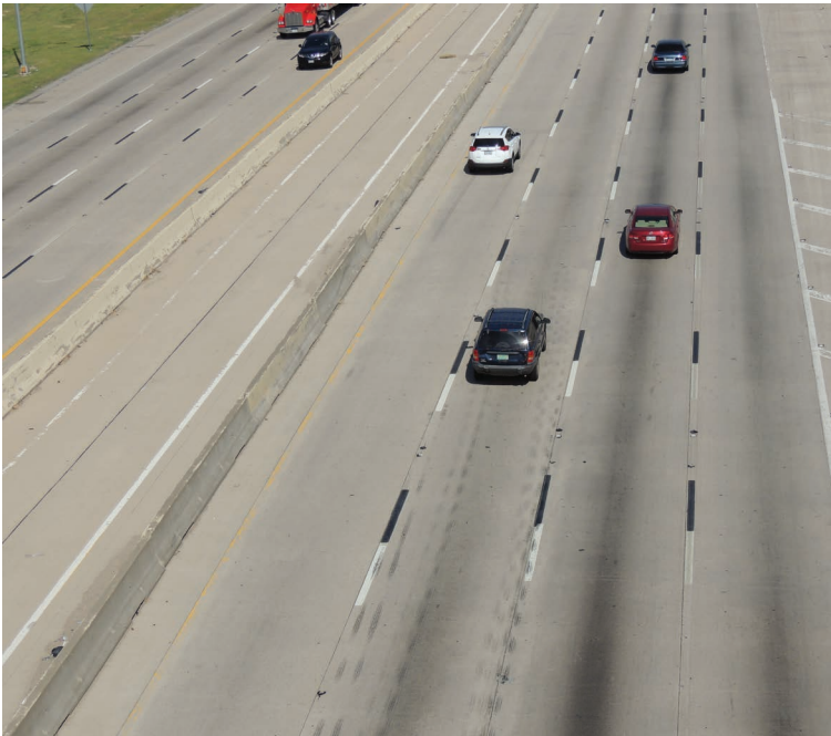
Figure 57. Contrast markings on light colored pavement
