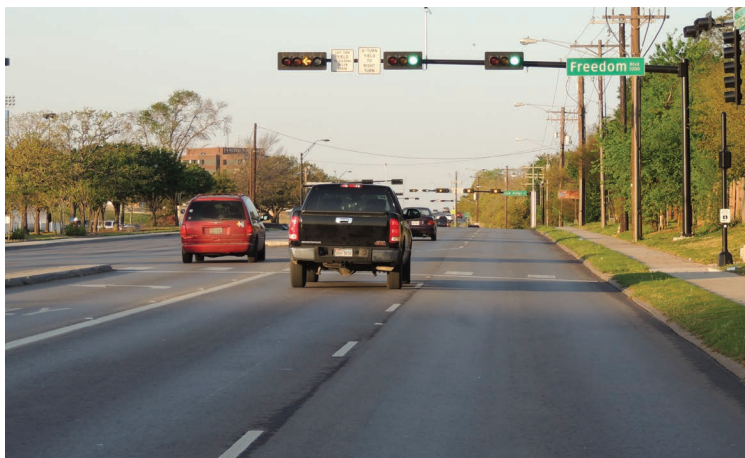
Figure 35. Example Of One Signal Head Per Lane
