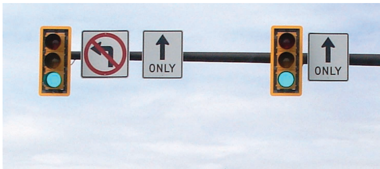
Figure 24. Yellow retroreflective backplates
