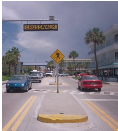
Figure 11. Raised median island with yellow marking on the vertical face and top surface
