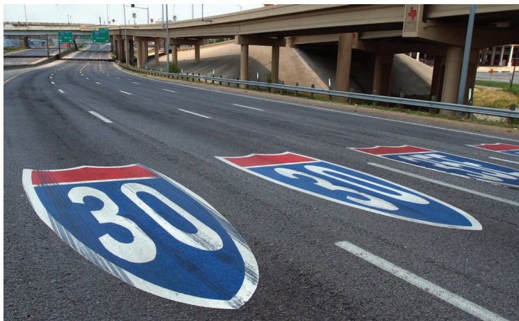
Figure 50. Route Shield Markings At Freeway Junctions
