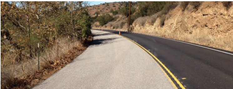
Figure 60. High friction surface treatment on a horizontal curve
