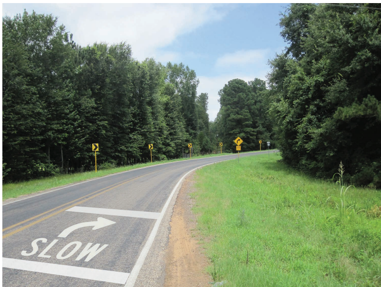
Figure 58. Curve warning markings (MUTCD:5)
