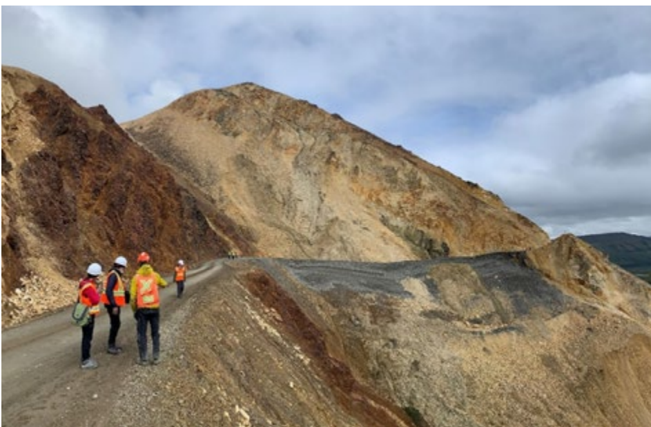
Field crews from the Western Federal Lands Highway Division visit the Pretty Rocks landslide to scope potential remedies for the land glacier as seen on the right side of the photo extending from the road into the valley below.
