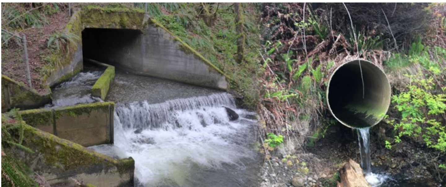
These two “perched” (outlet higher than the streambed) culverts may act as barriers to AOP, thereby disrupting long-stream connectivity and habitat functions of a river or stream. Fish trying to swim upstream would likely be unable to navigate the jump heights and the shallow water depths in the culverts.
