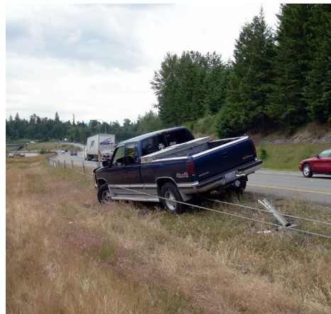
Median cable barrier prevents a potential head-on crash. Source: Washington State DOT
