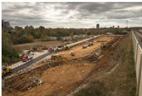
The NPEP mitigation area under construction. The noise wall can be seen on the right. The difference in elevation due to added fill can be seen in the center of the photograph.
