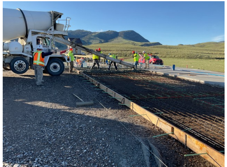
Concrete pavement pour north of the entrance station building and kiosks.
