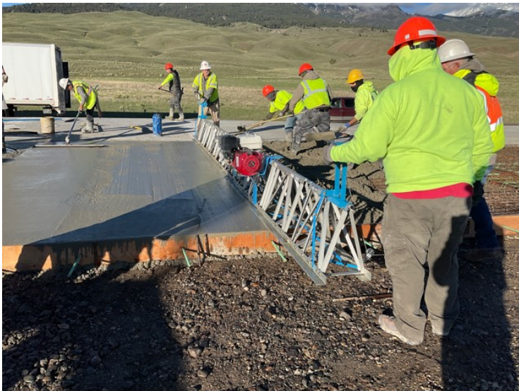
Concrete pavement pour north of the entrance station building and kiosks.
