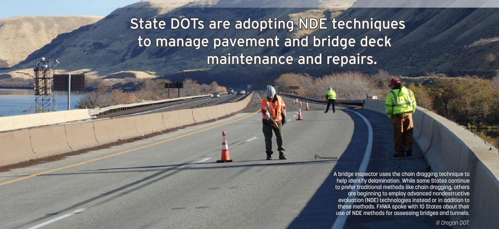
A bridge inspector uses the chain dragging technique to help identify delamination. While some States continue to prefer traditional methods like chain dragging, others are beginning to employ advanced nondestructive evaluation (NDE) technologies instead or in addition to these methods. FHWA spoke with 10 States about their use of NDE methods for assessing bridges and tunnels.
