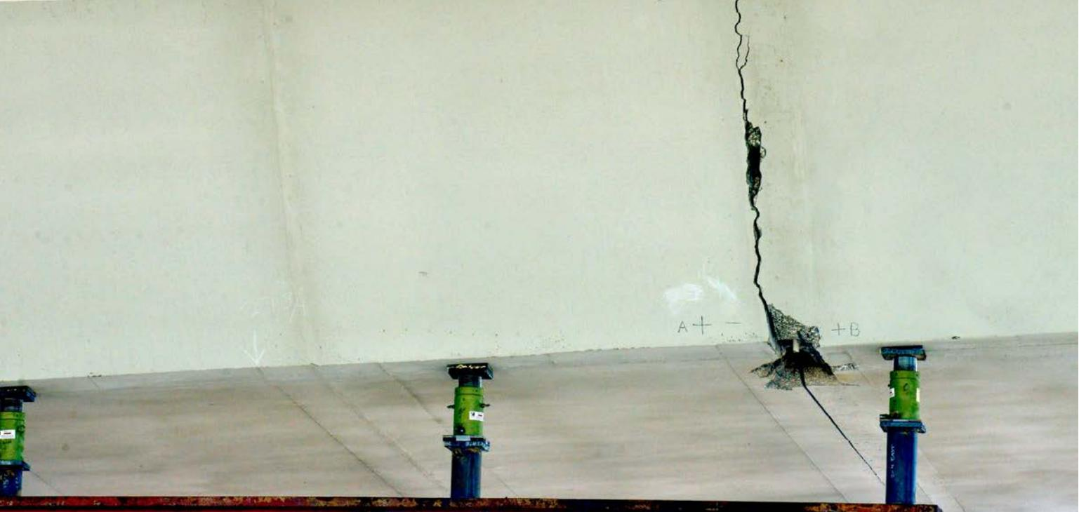
In June 2020, an inspection of the temporarily closed Roosevelt Bridge in Florida revealed corrosion and ruptured steel strands. Shown here is the exterior view of the damaged location.
