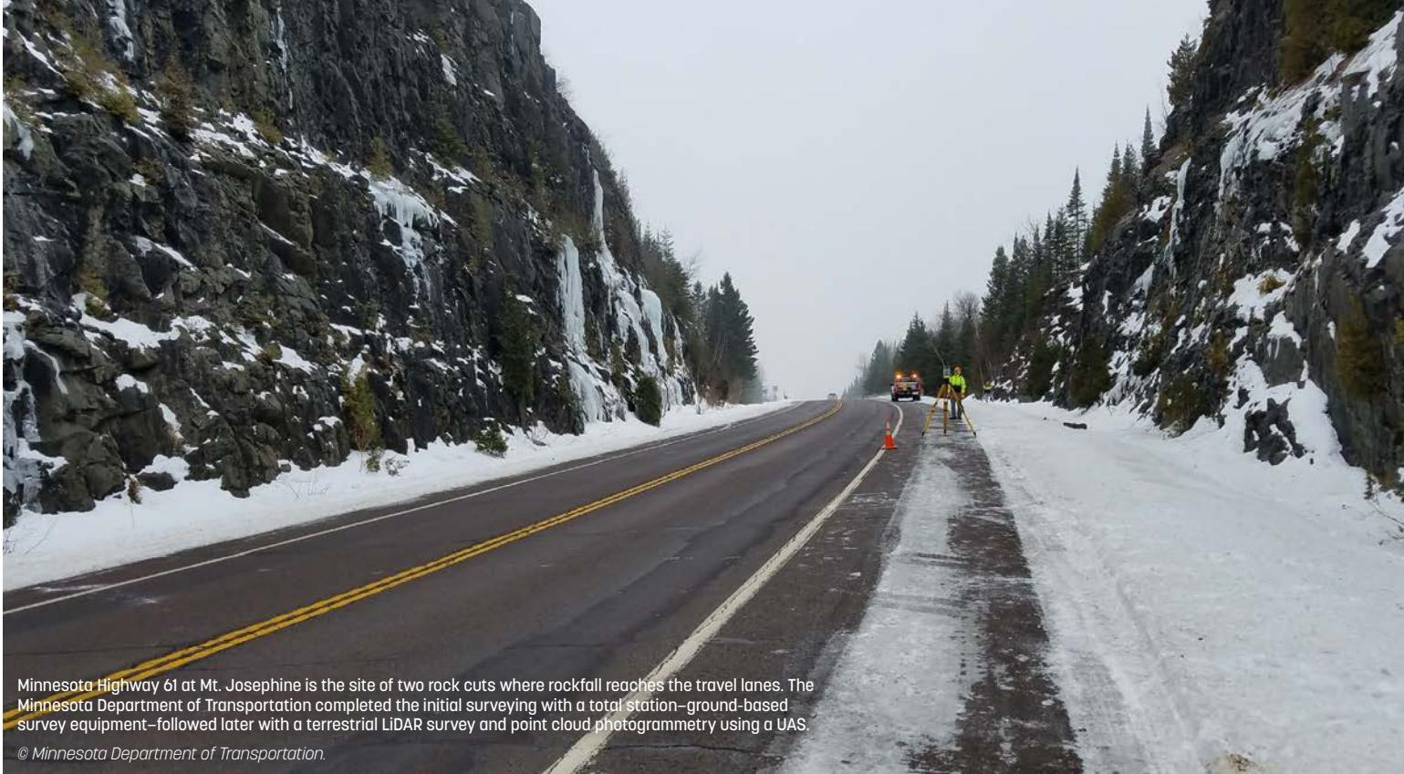
Minnesota Highway 61 at Mt. Josephine is the site of two rock cuts where rockfall reaches the travel lanes. The Minnesota Department of Transportation completed the initial surveying with a total station—ground-based survey equipment—followed later with a terrestrial LiDAR survey and point cloud photogrammetry using a UAS.
