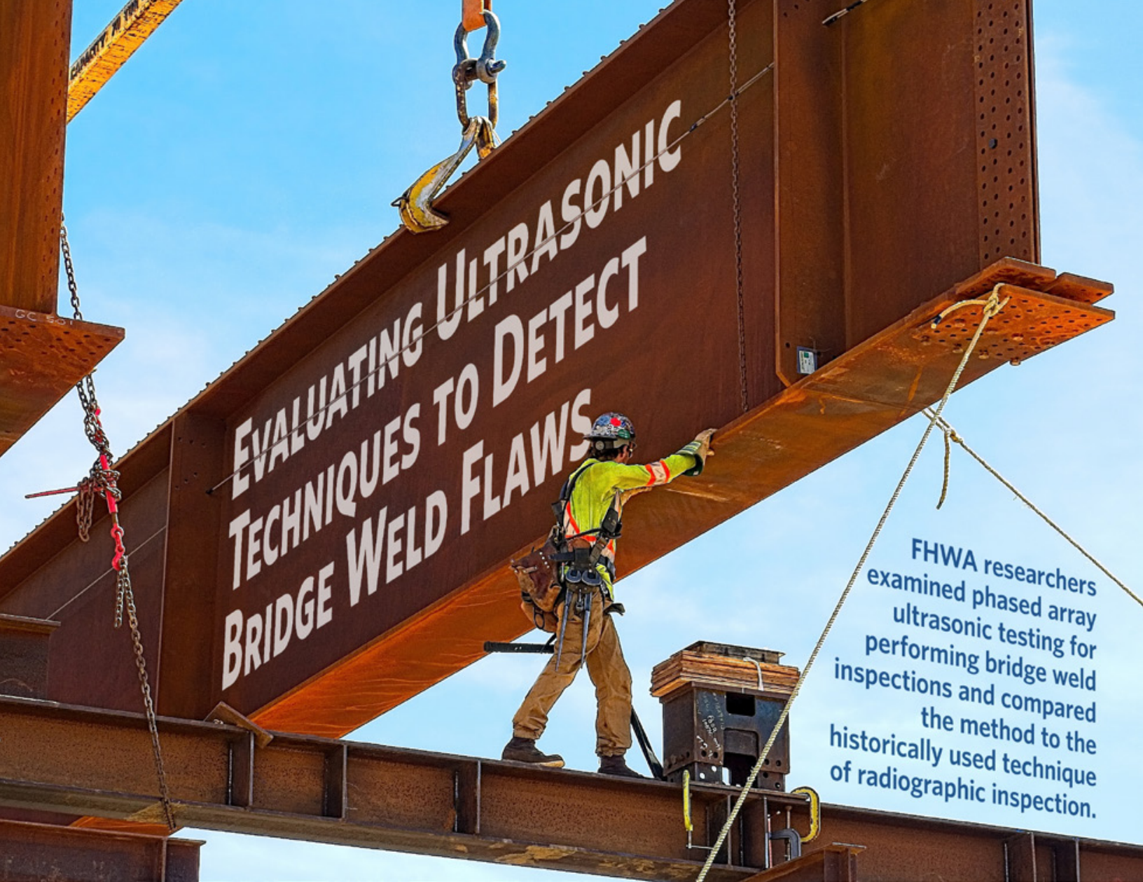
The welds between steel plates on bridge girders are critical to the strength and integrity of the bridge. Advances in nondestructive evaluation techniques like ultrasonic testing may help both manufacturers and field inspectors identify and address flaws safely and accurately.
