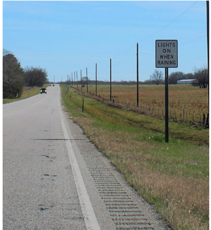
Rumble strips are effective for keeping vehicles in their lanes. Widening shoulders provides space for vehicle recovery and can also provide room for rumble strips.
