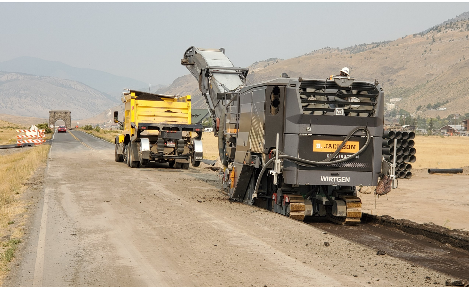
Milling Operation on North Entrance Road
