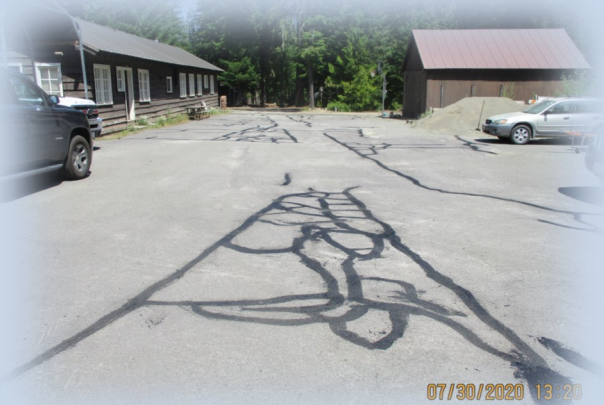
Crack Sealed Parking Lot at White River Ranger
