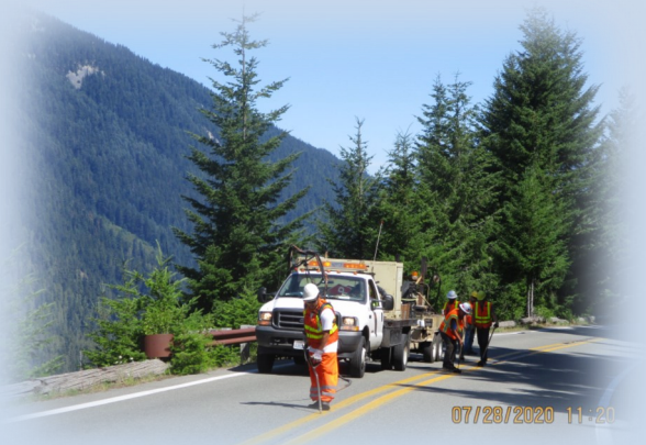
Crack Sealing on SR410
