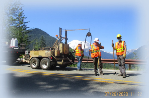
Crack Sealing on SR410 in shadow of Mt Rainier
