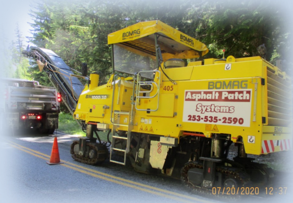
Milling and Removing the Old Asphalt
