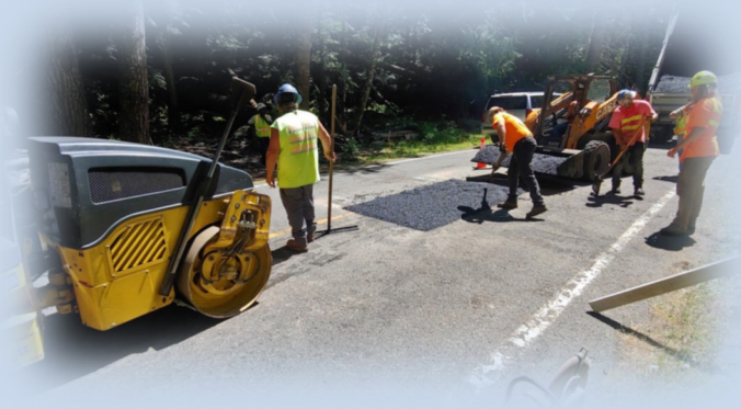
Placing Asphalt
