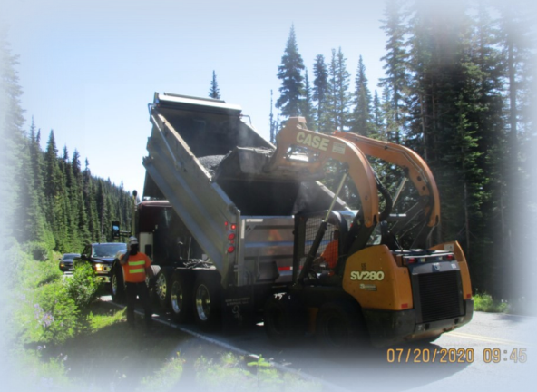
Dipping into the truck to get new Asphalt
