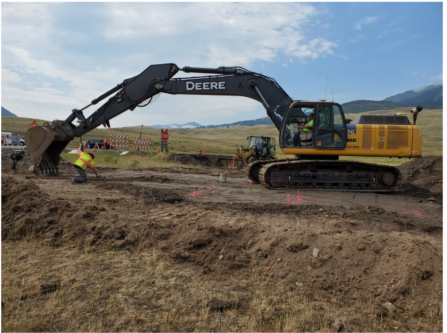
Foundation preparation for the main building.
