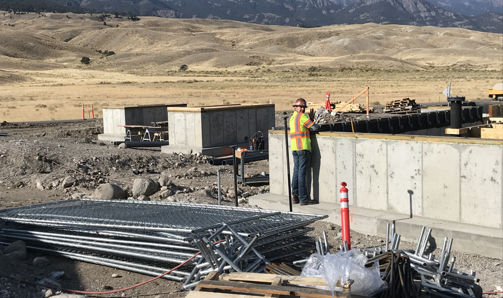
Stem walls poured and floor joists going in
