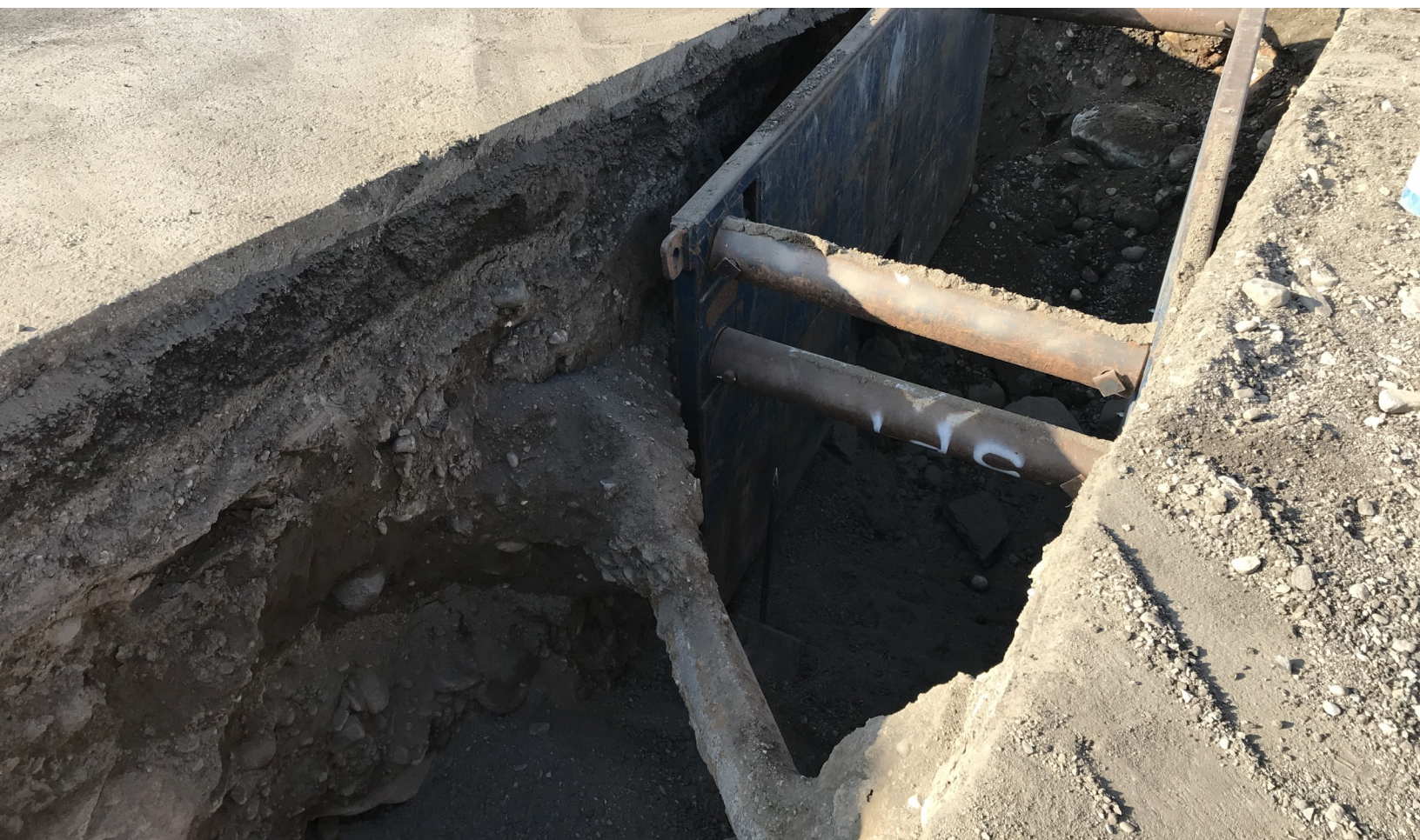
Trenchbox sitting next to existing waterline
