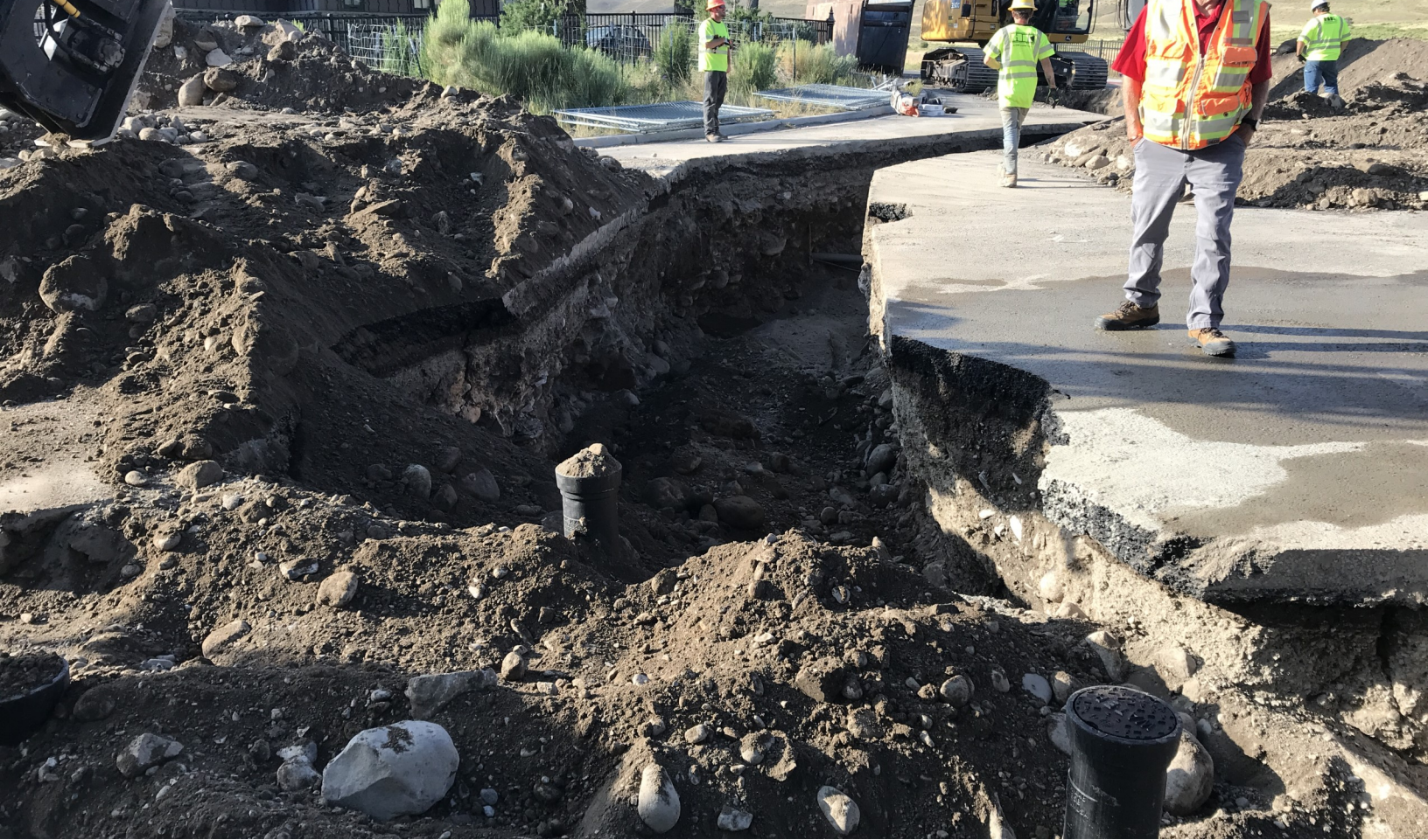
Waterline Tie in at Park and Rober Reamer Intersection. Valve boxes installed
