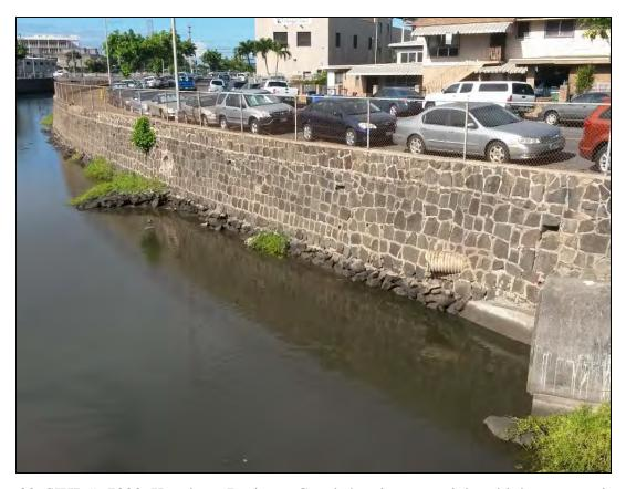
Figure 32. SIHP # -7808, Kapālama Drainage Canal showing potential multiple construction phases of the canal walls, view to southwest
