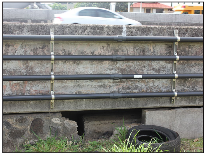
Photo 4. Gaps in the concrete beneath H-1, Mauka side of the bridge
