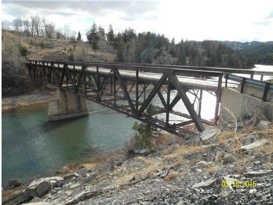
PHOTO #1 MTA-SR-001, SUN RIVER BRIDGE, PHOTO BY GARY GRASSEL. VIEW LOOKING AT THE UPSTREAM SIDE OF THE BRIDGE. (03/18/2015)
