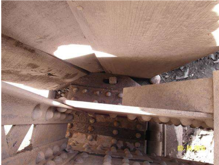
PHOTO #13 MTA-SR-001, SUN RIVER BRIDGE, PHOTO BY GARY GRASSEL. THIS IS A VIEW OF THE UPSTREAM SIDE AT THE SAME APPROACH AS IN PHOTO #12. THE ANCHOR BOLT IS BENT AND THE BEARING PLATE HAS EXTENDED PAST THE FIRST ROLLER. (03/18/2015)
