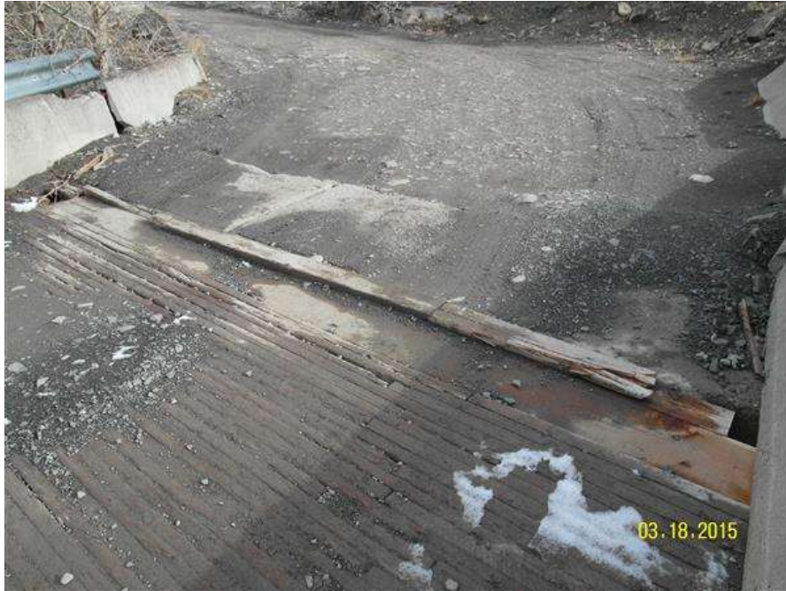
PHOTO #5 MTA-SR-001, SUN RIVER BRIDGE, PHOTO BY GARY GRASSEL. THIS PHOTO SHOWS THE LEFT (EAST) APPROACH SPAN OF THE BRIDGE. REPAIRS HAVE BEEN MADE SINCE THE LAST INSPECTION. (03/18/2015)
