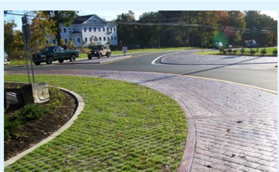
After: Close-up of truck apron constructed during conversion to roundabout, along with a raised truck “blister” on the outside of the roundabout.
