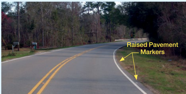
Example of 20 feet RPM spacing for a curve.
