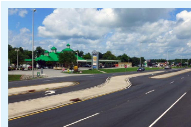
Restricting the direct crossing movement reduces the number of conflict points and severity of crashes.
