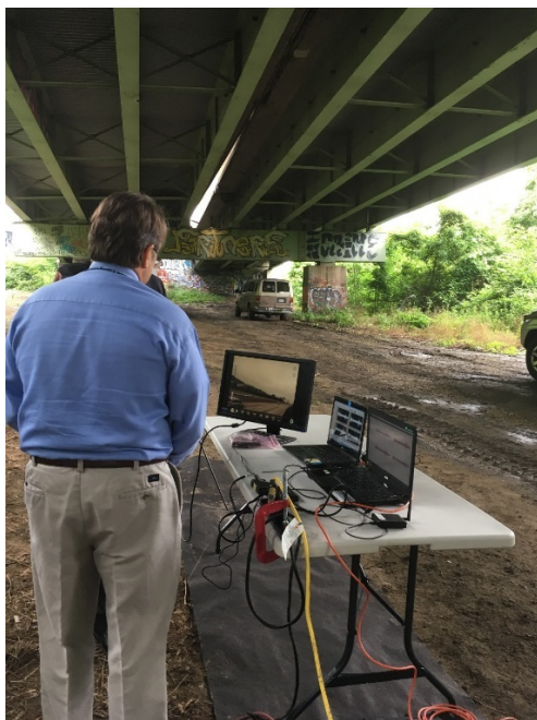
A researcher monitors the computer displays of data received from wireless sensors installed on the roadway bridge during a demonstration as part of a TRL Assessment. (Source: U.S. DOT-owned)
