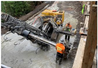
Photo left: Shows Drilling Ground Anchors at MP 56. All images Source: FHWA
