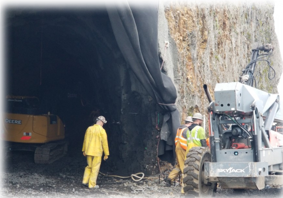
Below Right: West tunnel portal drilling
