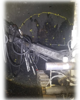
Left: East portal pattern of blast
