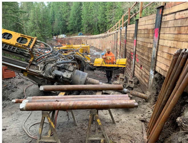
Photo left: Shows Drilling Ground Anchors at MP 56. All images Source: FHWA
